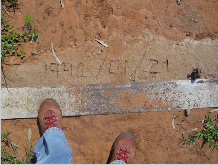
Fig.9 A date of 21/01/1994 confirms when the feature was constructed.
