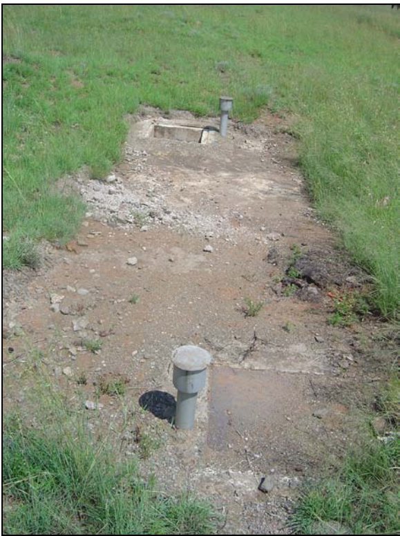
Fig.12 Part of the existing sewer installation in area B.
