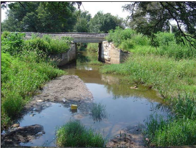
Fig.6 The railway bridge across the main flood furrow from Uitsig.
