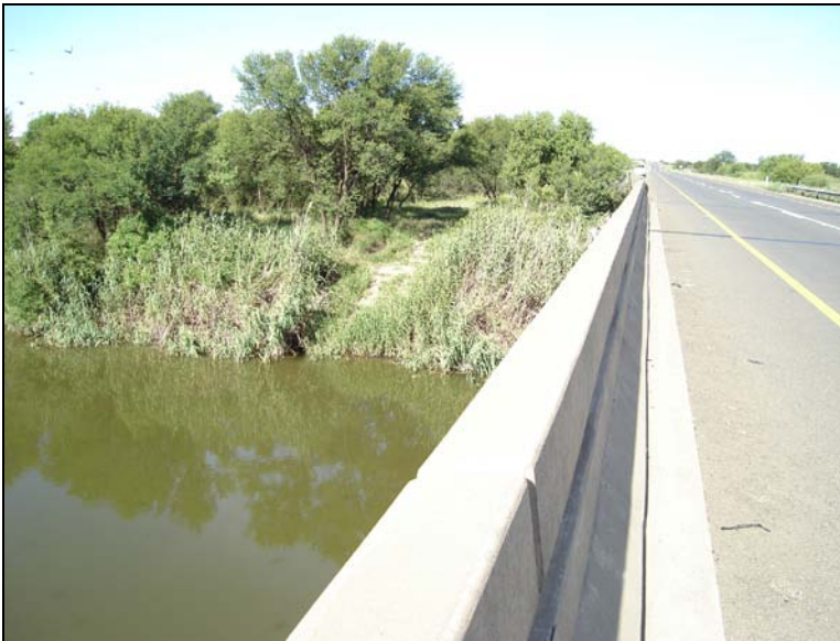
Fig.5 Bridge on the Renoster River on the N1.
