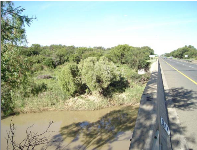
Fig.7 Bridge on the Modder River along the N1..
