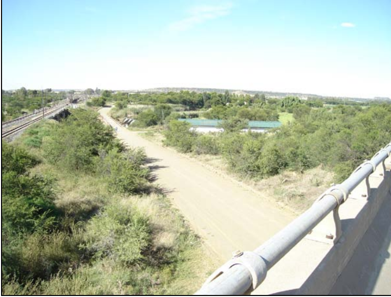
Fig.6 Railway bridge at Renoster River N1.
