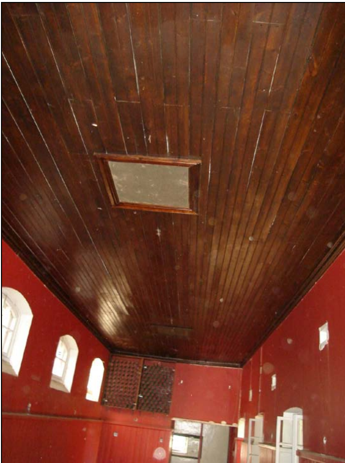
Fig.10 Detail of the interior ceiling of the stables.
