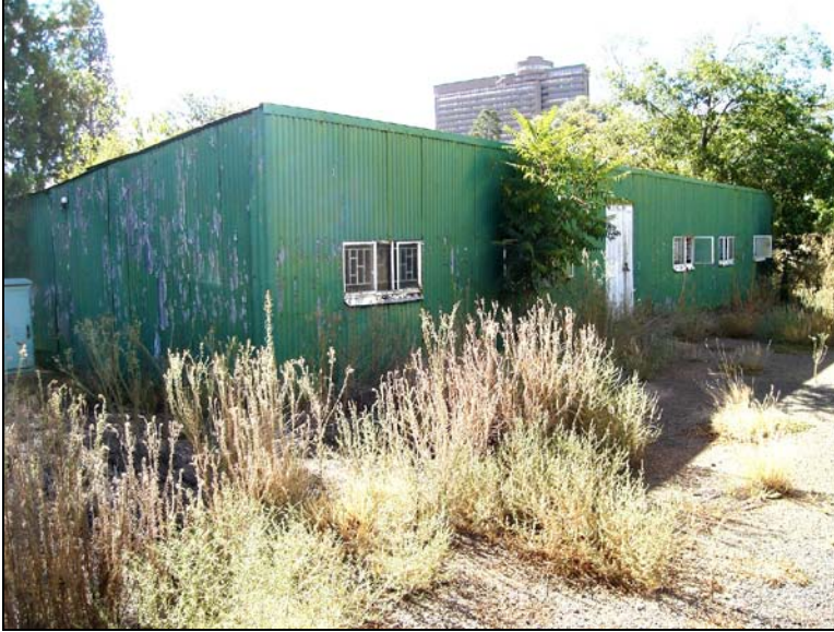
Fig.43 Corrugated iron shed near the water reservoir at point C.
