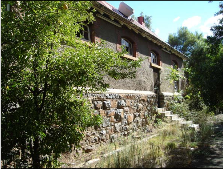
Fig.11 North wall with kitchen back entrance.
