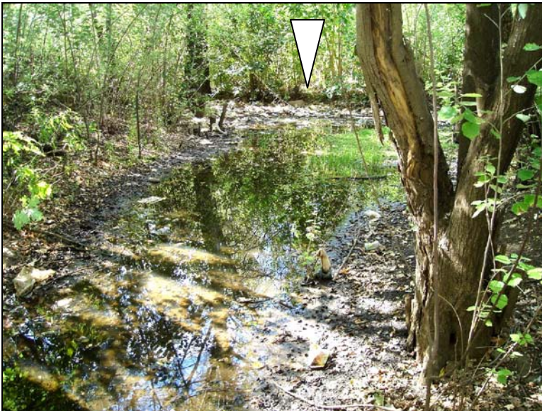
Fig.52 Rainwater forms a permanent pool against the old dam wall.
