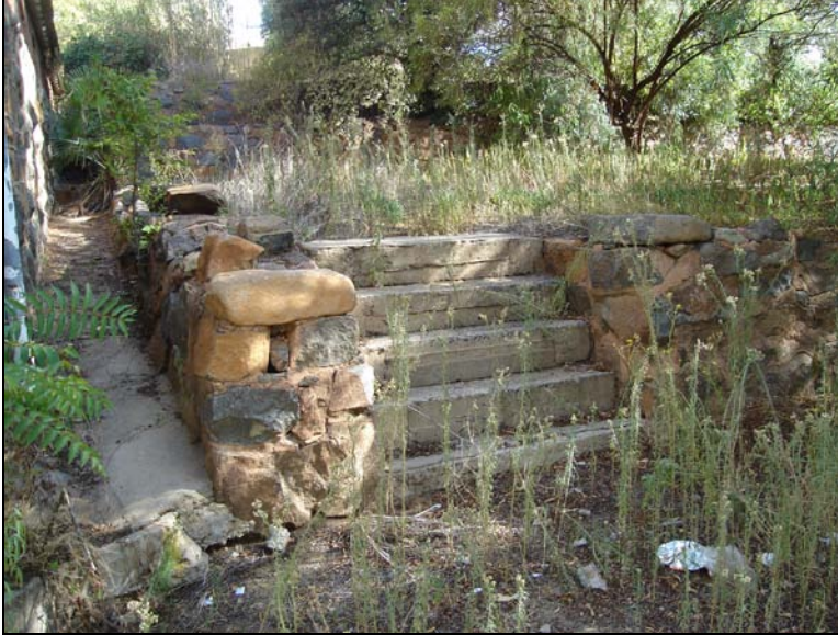
Fig.45 Concrete steps and stone terrace walls behind the kitchen (stables).
