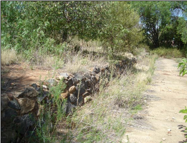
Fig.50 Dolerite terrace wall near large concrete slab.
