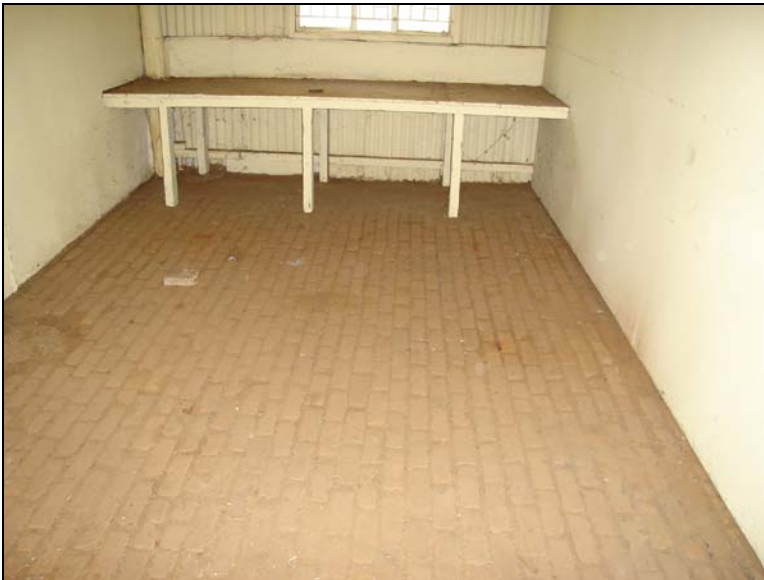
Fig.44 The original brick paved floor of the shed is still intact.
