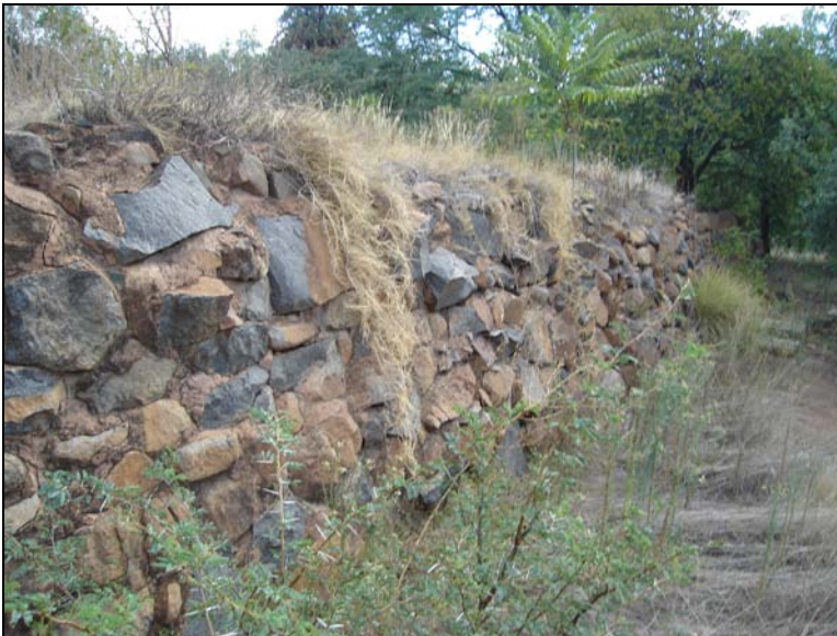
Fig.46 A very prominent stone terrace wall behind the stables
