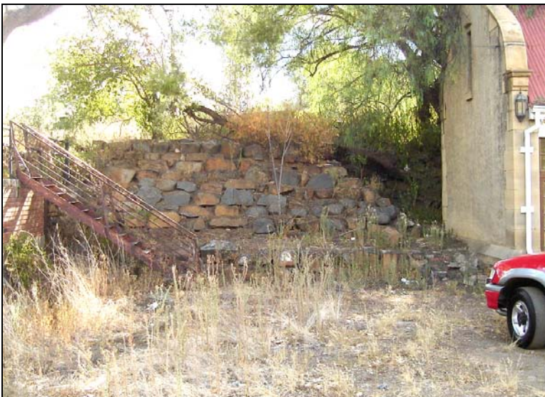
Fig.48 Stone-walled terrace next to and running behind the stables.
