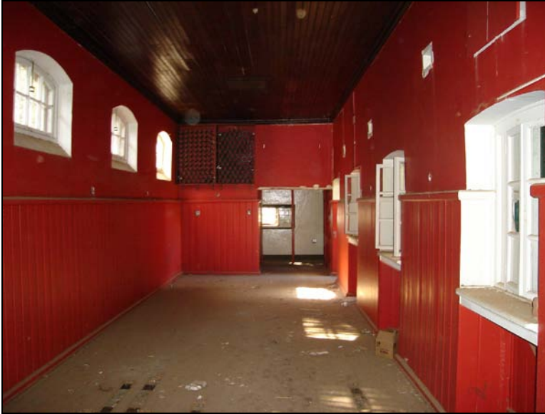
Fig.9 Interior of the Stables facing towards the kitchen.
