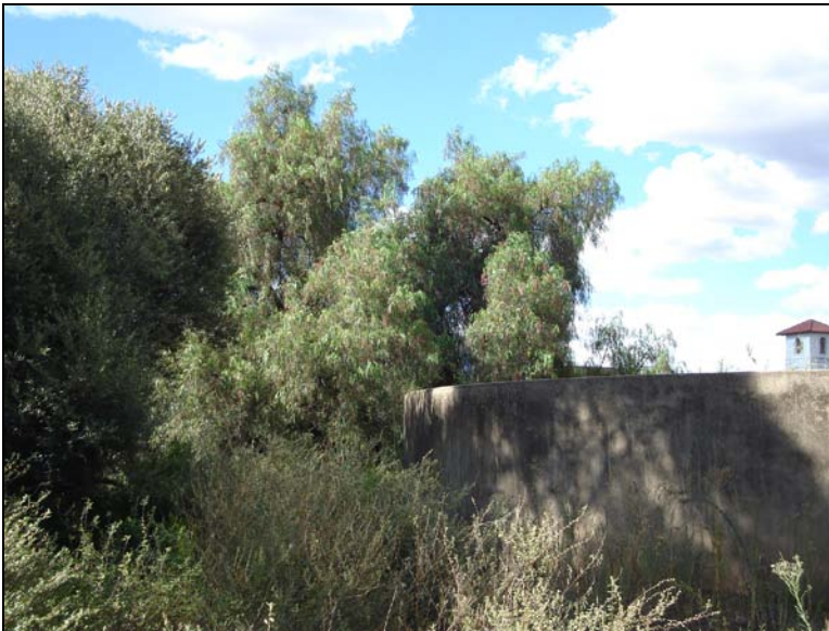
Fig.18 Point C near the water reservoir dam.
