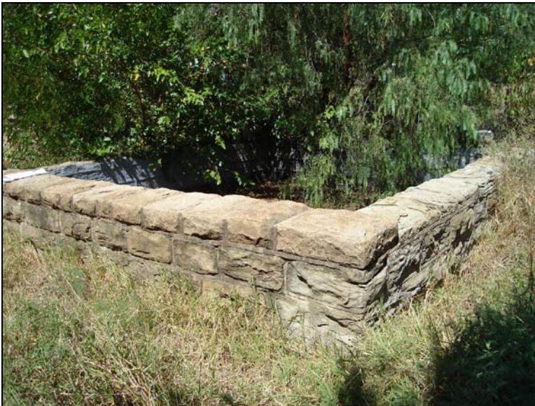
Fig.14 Reservoir dam 1, allegedly built during the time of Pres. Reitz (1889-1895).
