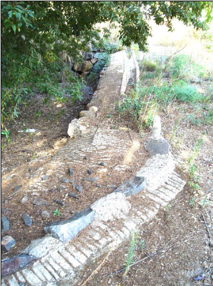
Fig.54 Concrete paving and irrigation furrow.
