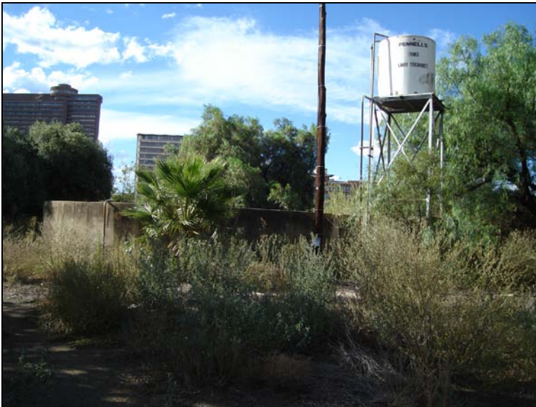
Fig.36 Water reservoir dam 2 and tank installation at the borehole.
