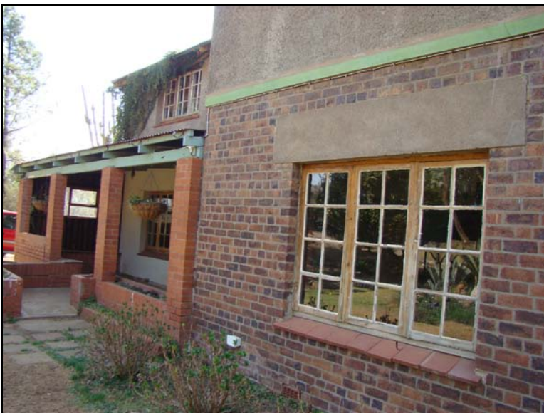
Fig.9 Front view of the old house as seen from the east.
