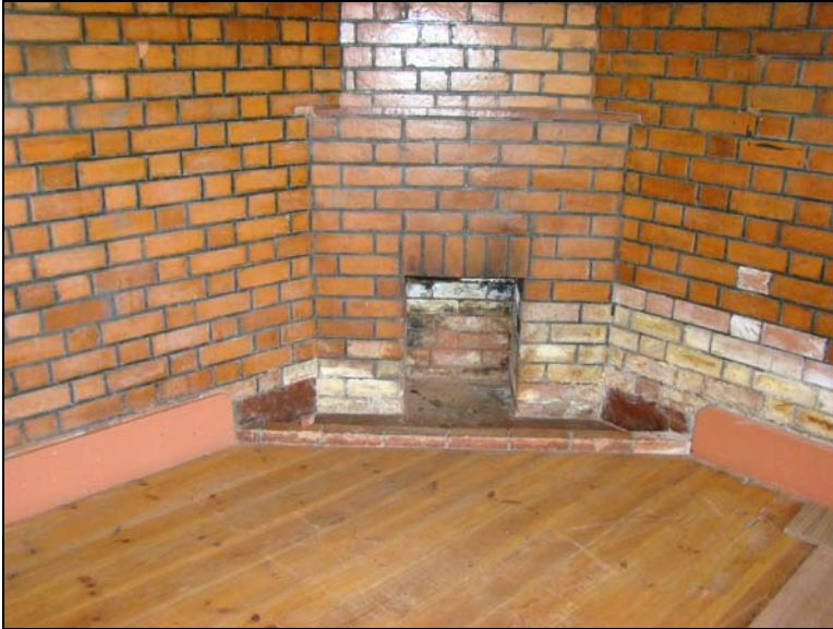
Fig.19 Fire place in the dining room.
