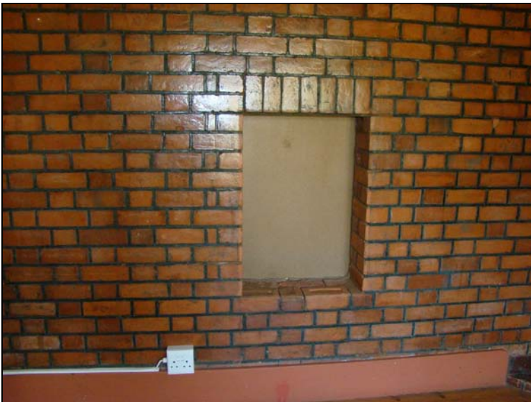
Fig.20 Service opening between the dining room and kitchen.
