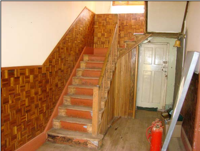
Fig.17 Staircase leading to the first floor.
