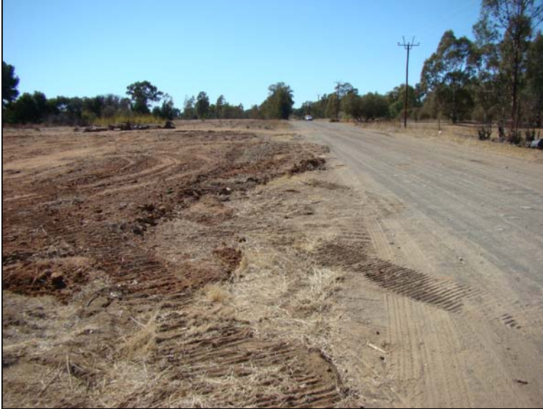
Fig.6 View from Point D facing along Eland Avenue towards Point A.
