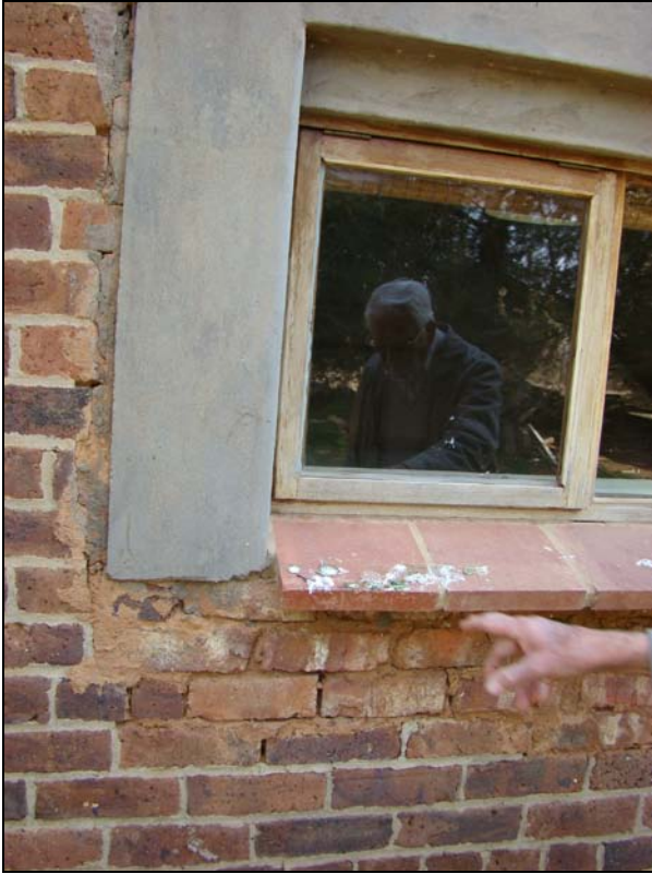
Fig.14 Lower window on east side had been replaced previously.
