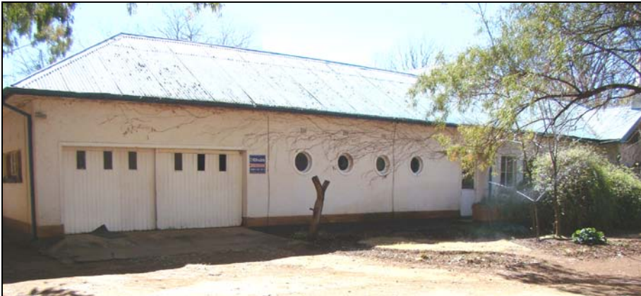
Fig.18 The south eastern part of the house does not match the original style and seems to be a later addition.
