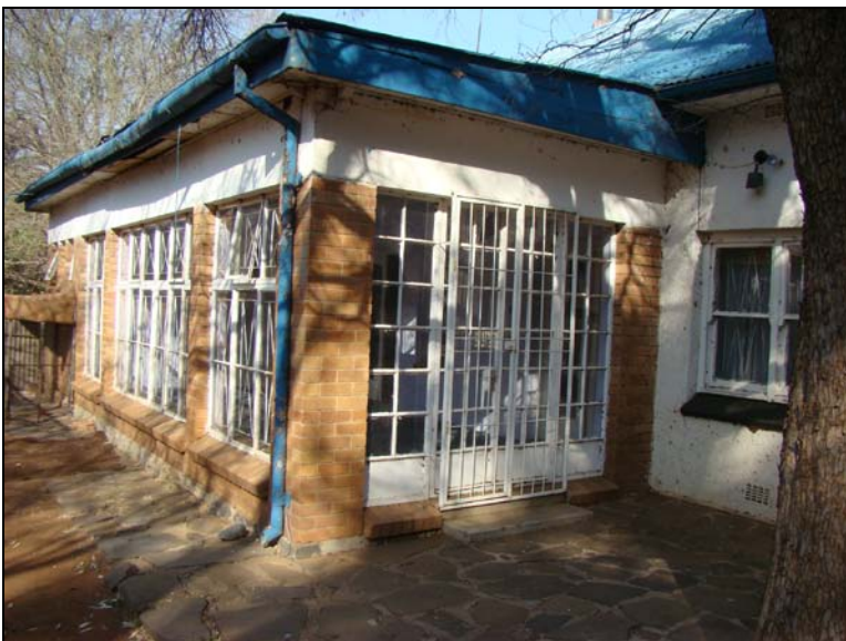
Fig.19 A sun porch on the western side of the house. This also does not match the original style.
