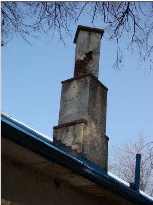
Fig.17 A smokestack at the farmhouse. The outer surface is finished in rough cast plaster.
