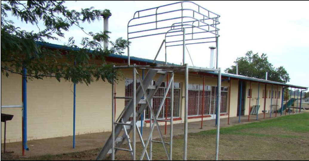
Fig.16 Rear view of the Club House at the Bloemfontein Equestrian Centre.
