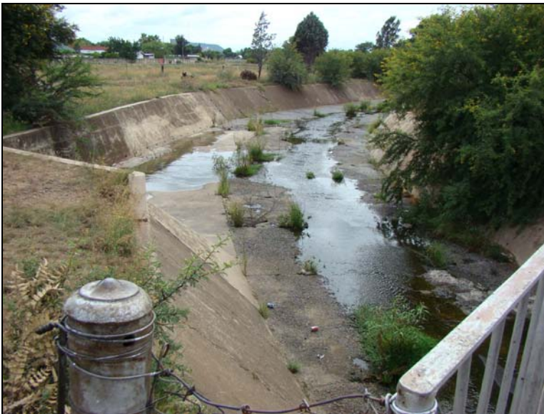
Fig.3 Point B facing east along the storm water channel.
