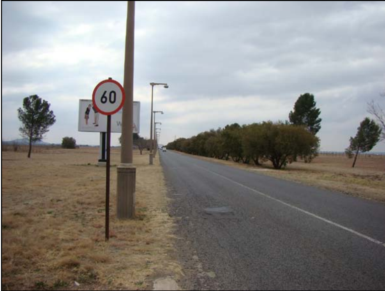
Fig.5 Point B facing the Bloemfontein Airport.
