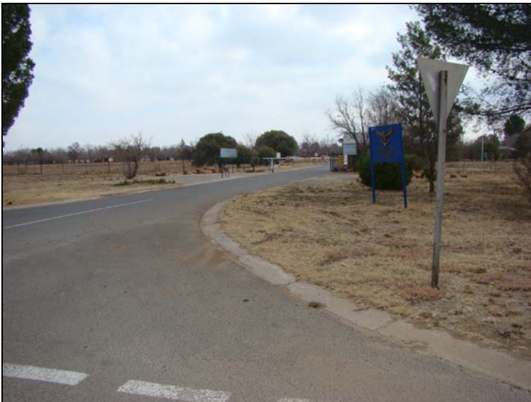
Fig.4 Pont B at the entrance to Bob Rogers Park.
