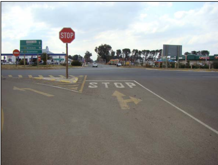
Fig.14 Point F at the N8 – filling station junction.
