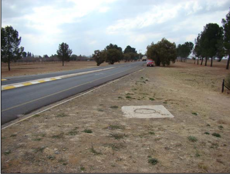
Fig.17 Point G at the N8 – Airport entrance junctin.
