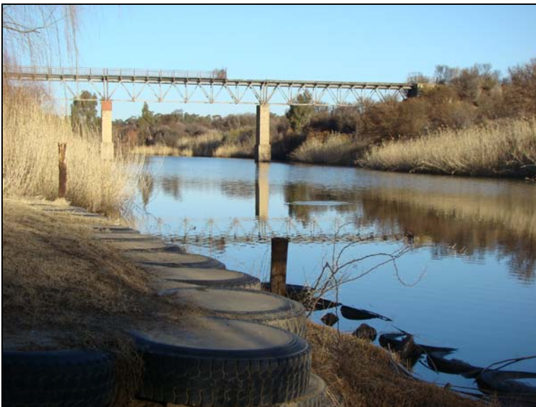
Fig.9 Old bridge across the Modder River on the way to Verkeerdevlei.
