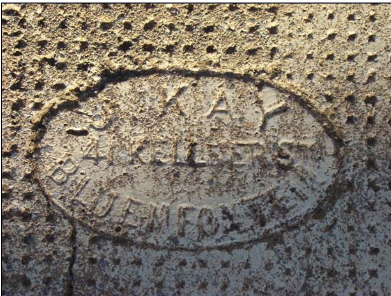
Fig.10 Badge of the manufacturer on the bridge. J. Kay, 41 Kellner St. Bloemfontein.
