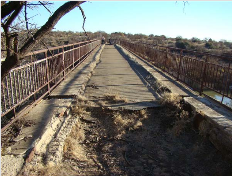
Fig.8 Old bridge across the Modder River on the way to Verkeerdevlei.
