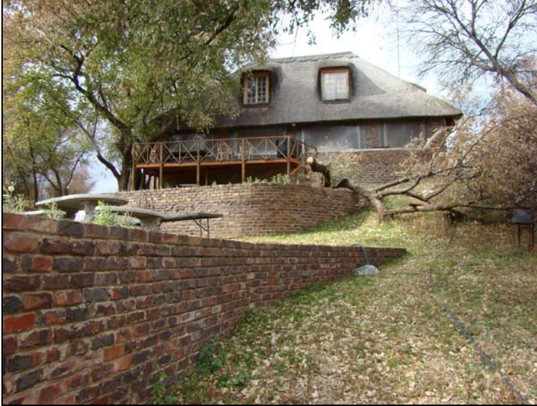
Fig.5 The existing river house.
