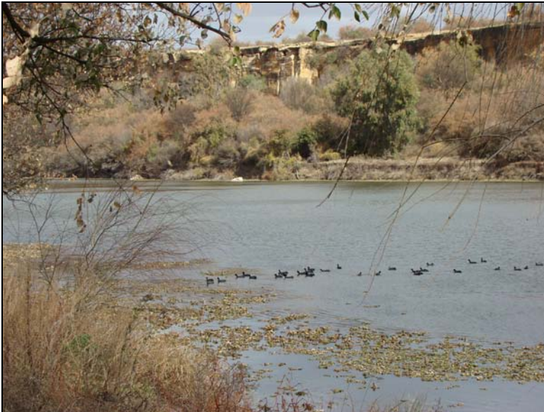
Fig.6 View across the stream at the river house. Note the solid cliffs on the opposite bank.
