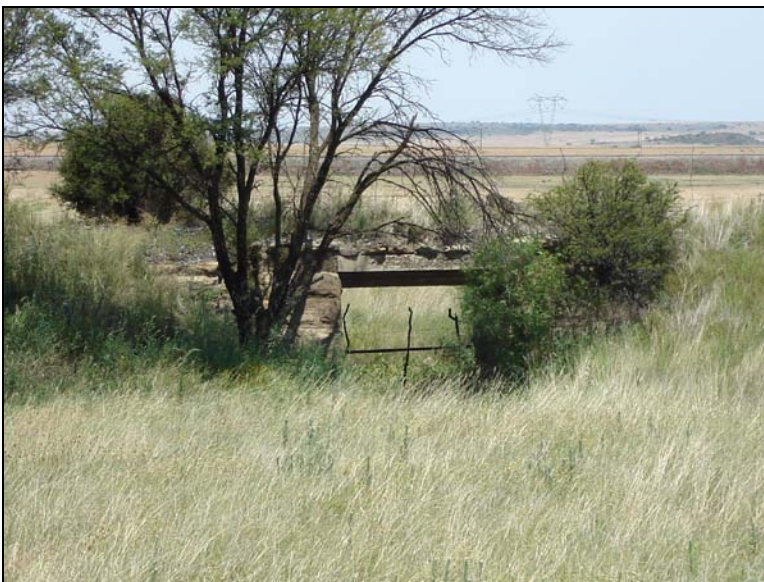
Fig.14 Old railway bridge near BP km 6,4 at Bella Vista.
