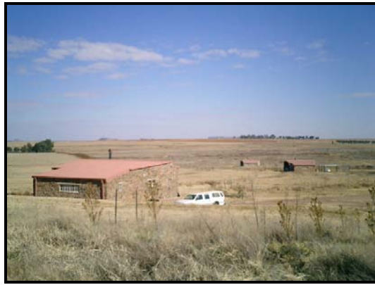
IMAGE 2: View from Spitskop over the existing development and proposed localities of units 4 and 5
