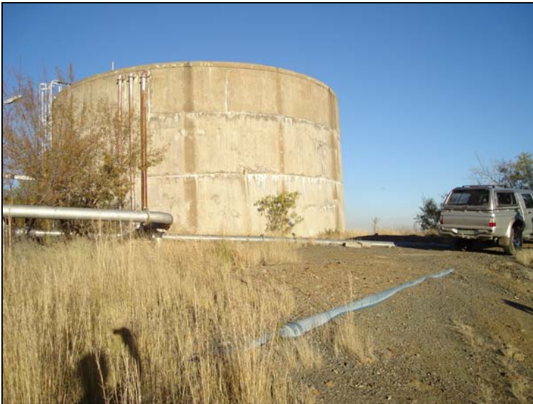
Fig.17 Water reservoir at Jagersfontein.
