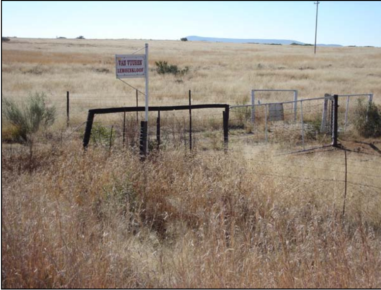
Fig.6 The road crossing at Lemoenkloof.
