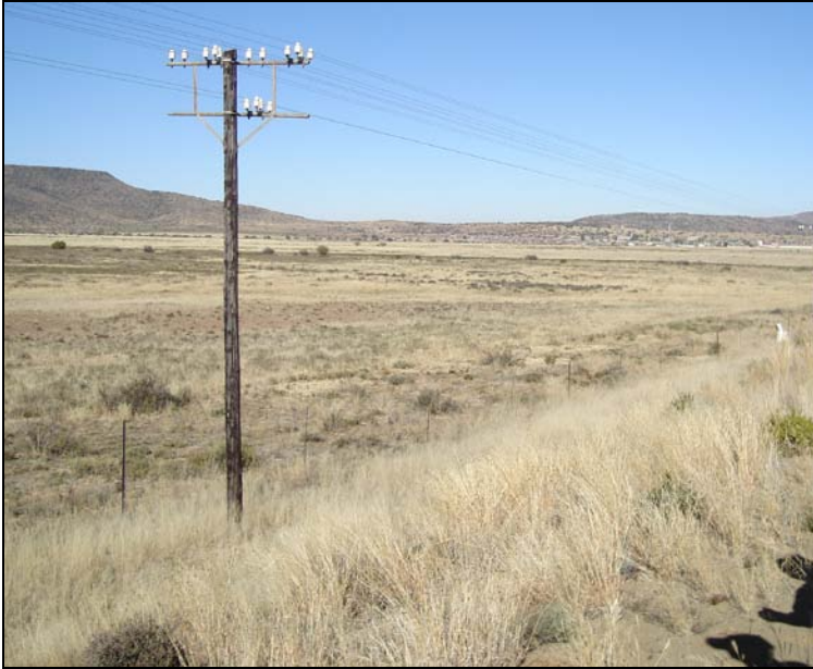
Fig.8 View along the pipeline route just before Fauresmith.
