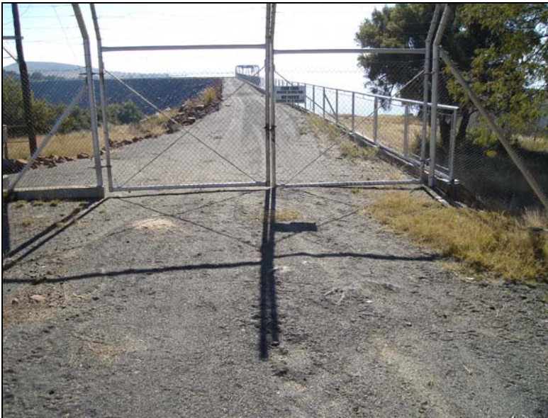
Fig.1 Kalkfontein Dam where the pipeline will start.
