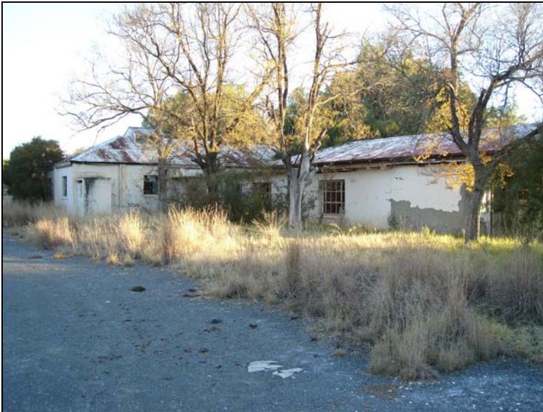
Fig.20 Another old and ruined building in the mining area.
