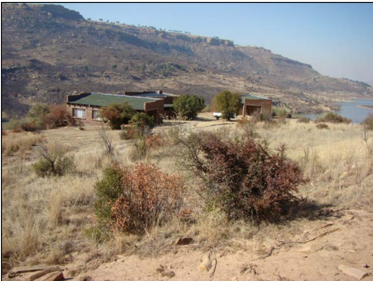
Fig.4 The Lodge at Point C facing towards the Meulspruit Dam.
