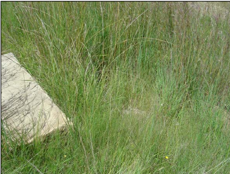
Fig.6 Old culvert indicates the position of the old road.
