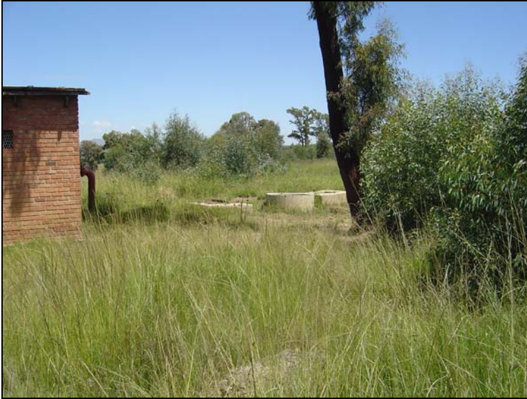
Fig.7 The pump house.
