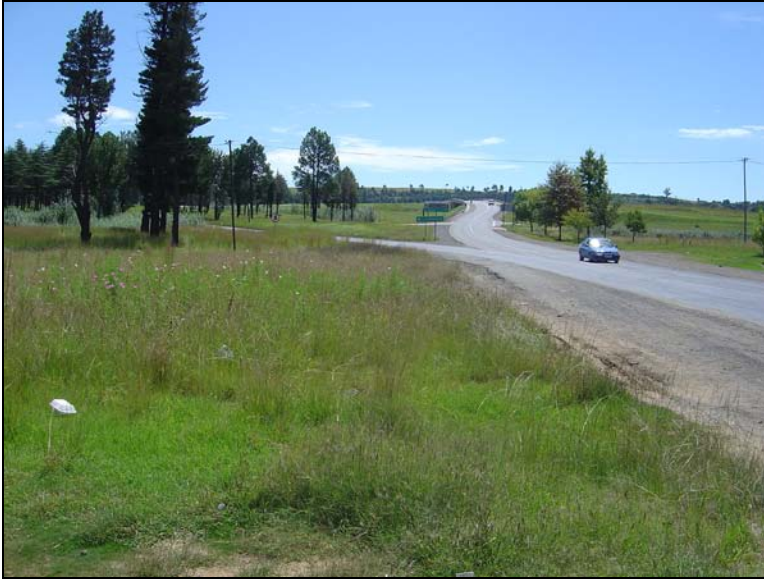
Fig.5 The spruit and the N3 junction.
