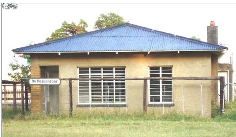
Fig.25 The old post office building is now part of the stock auction kraals.
