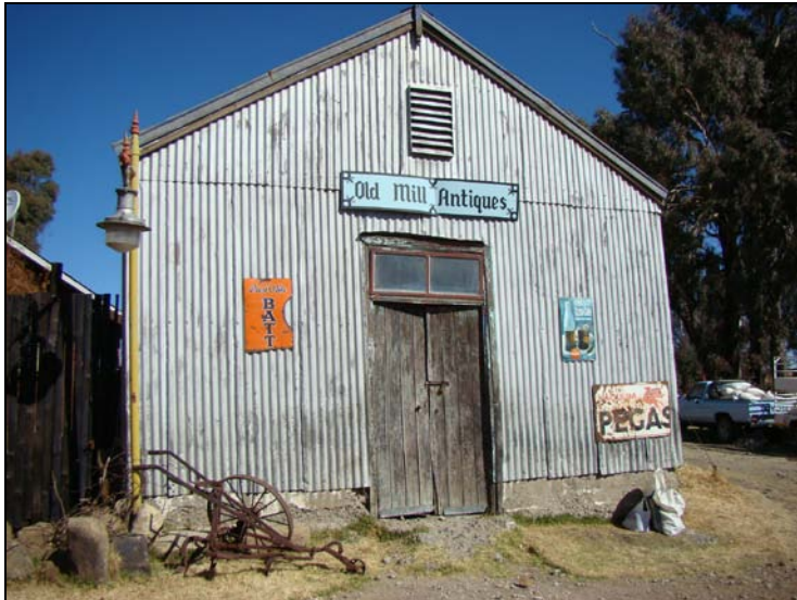
Fig.6 Façade of the old mill building.
