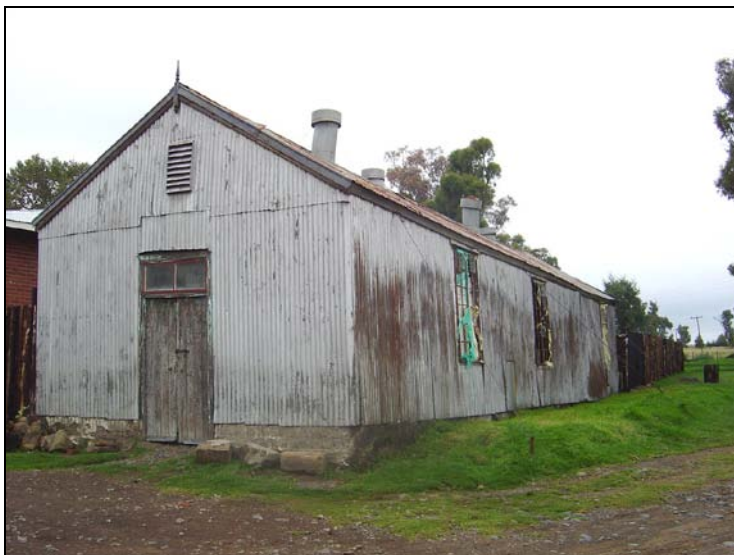
Fig.7 Front view of the old mill building.
