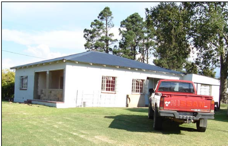
Fig.13 House adjacent to the general dealers' store.
