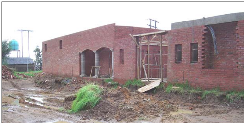
Fig.19 New SAPD buildings under construction.
