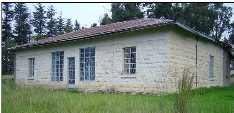
Fig.16 Painted sandstone house at Verkykerskop.
