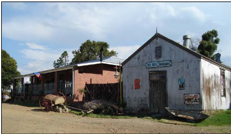
Fig.10 View of the old mill adjacent to the general dealers' store.
