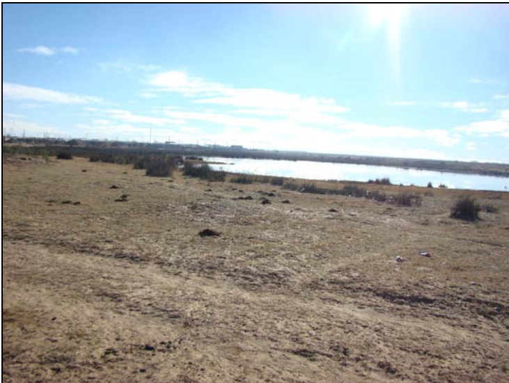
Fig.5 Point C facing west across the dam.
