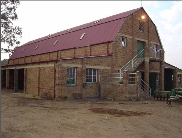
Fig.1 A north view of the building with northern annexure at Smaldeel, Kroonstad.
