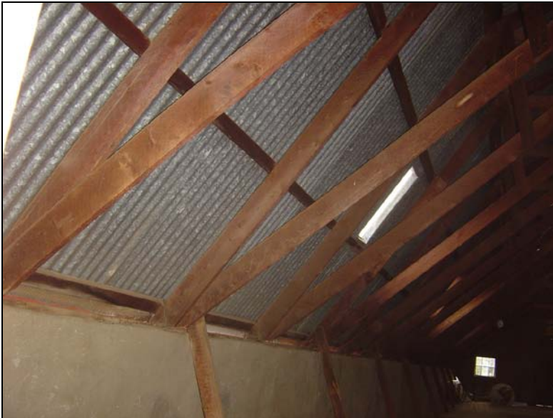
Fig.6 Detail of the roof of the barn at Smaldeel, Kroonstad.
