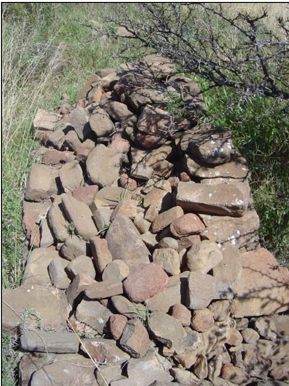
Fig.3 Remains of stone-walling indicating the building method with two sides and inner filling.
