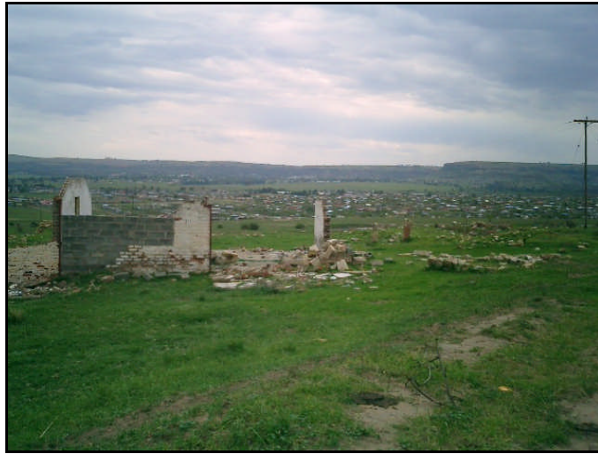
Figure 17: General view of the complex of outbuildings related to Site 1
