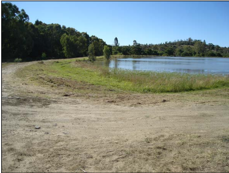
Fig.1 View from Point LDA across the existing reservoir dam at Lindley.
