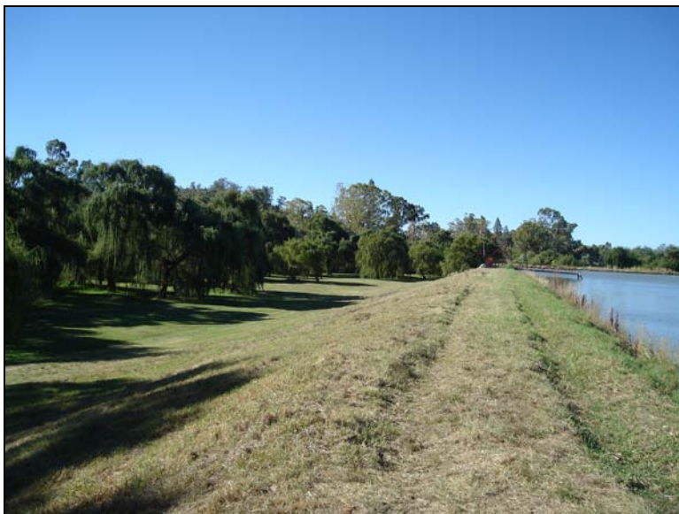
Fig.6 View along the existing reservoir dam wall.
