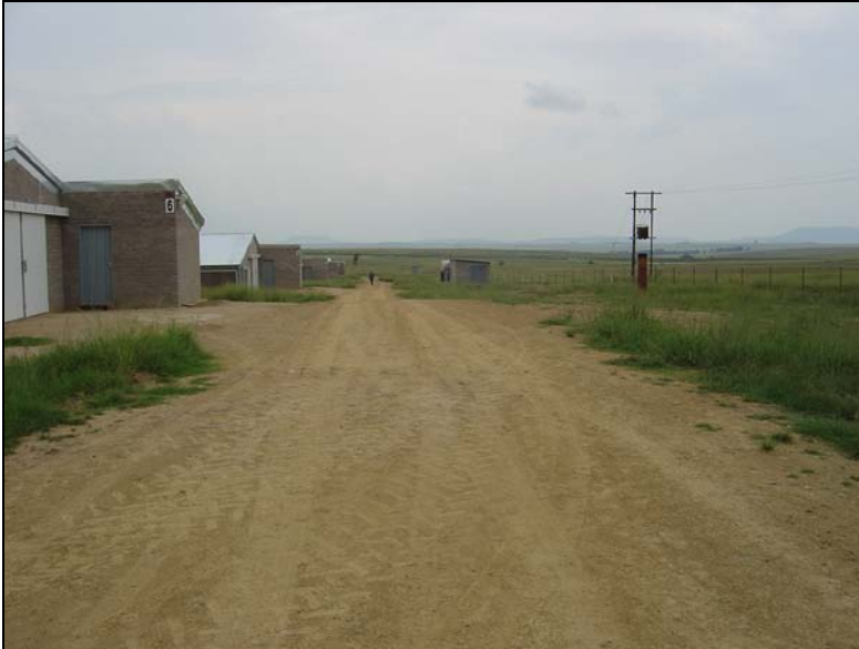
Fig.1 View of the existing chicken breeding installations at Vaalkoppies 215, Arlington.
