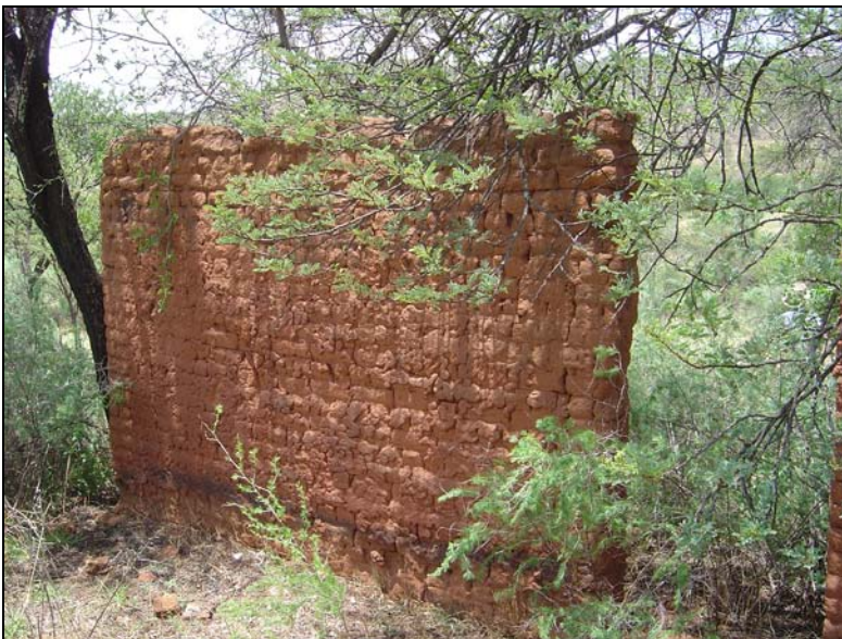
Fig.12 Unbaked clay brick wall of a pioneer house at Aasvogelrand, Vredefort
