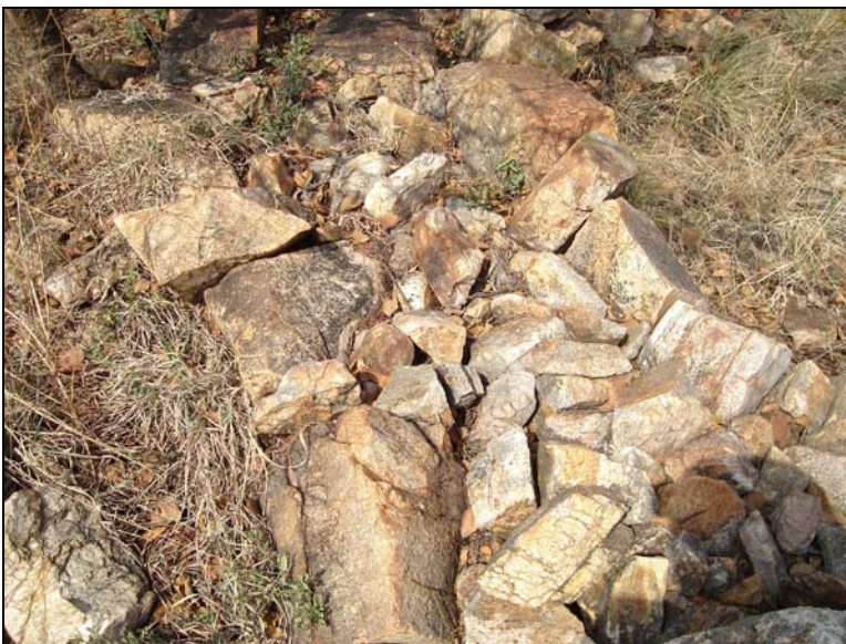
Fig.8 Stone-walls show the traditional building style of two separate outer walls with rubble infill in the centre.
