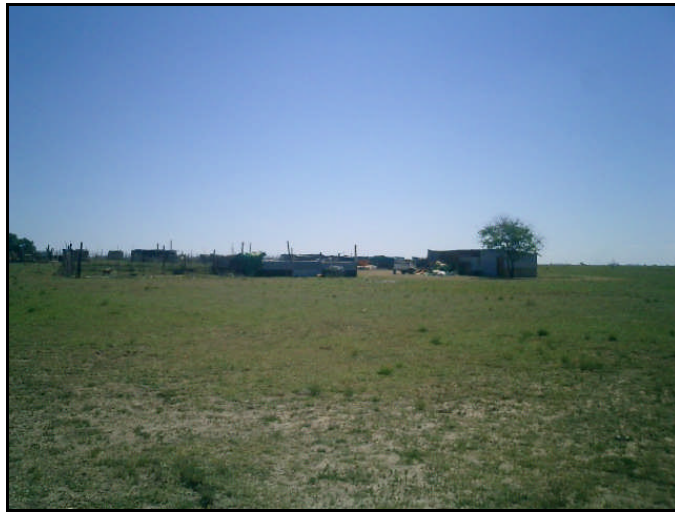
Figure 11: General view of Site T1's living quarters
