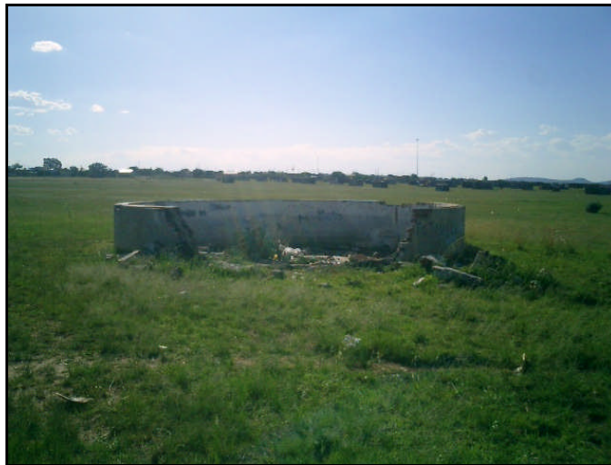
Figure 14: The Site T3 cement dam remains
