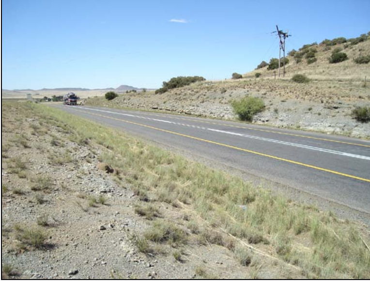
Fig.8 Road cutting at Km 39,0 on the N1 between Gariep Dam and Springfontein.
