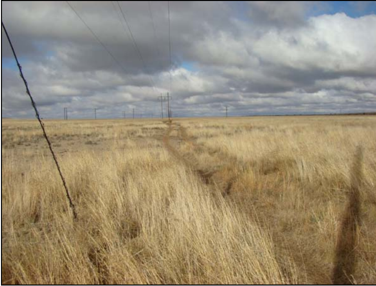
Fig.14 Pylon 17 on the Springfontein – Reddersburg line.
