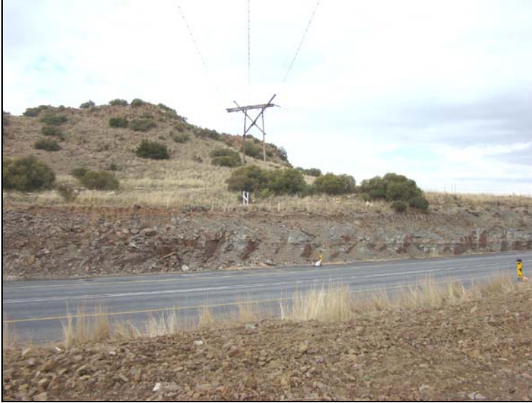
Fig.10 Oranjekrag – Springfontein line – N1 crossing.
