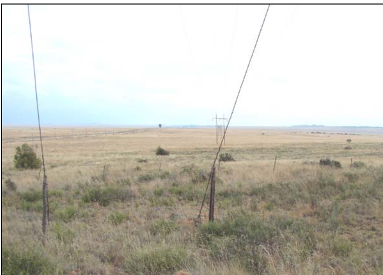
Fig.23 Pylon 101 on the Edenburg – Reddersburg line.
