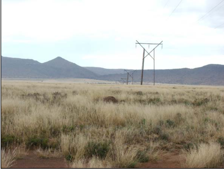
Fig.4 View from Pylon 32 on the Oranjekrag – Springfontein line.
