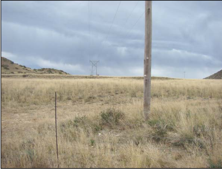
Fig.8 Pylon 153 on the Oranjekrag – Springfontein line.
