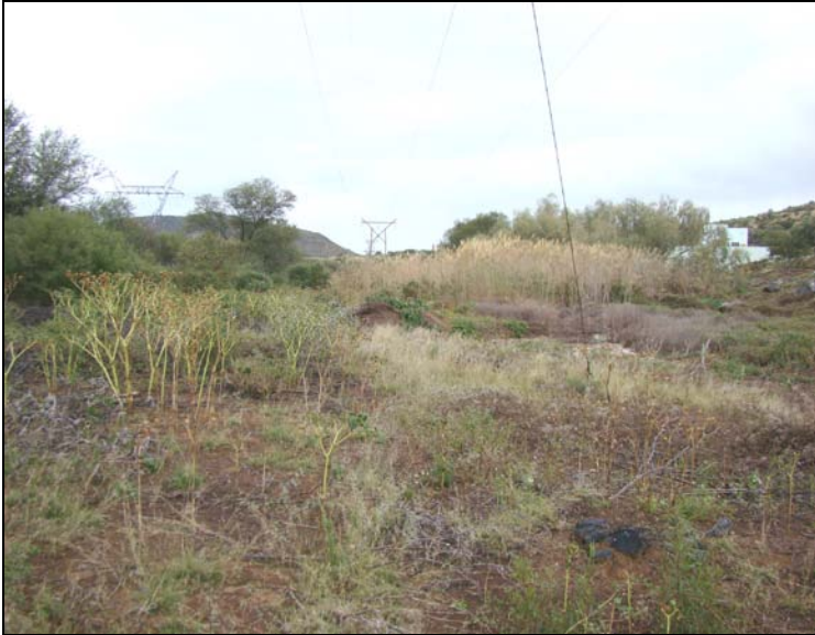
Fig.2 Pylon 14 near Oranjekrag Sub-station.
