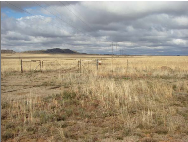
Fig.15 Pylon 53 on the Springfontein – Reddersburg line.
