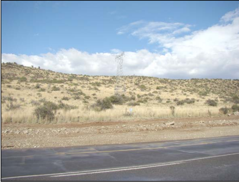
Fig.6 Power line on the Oranjekrag – Springfontein sector along the N1.
