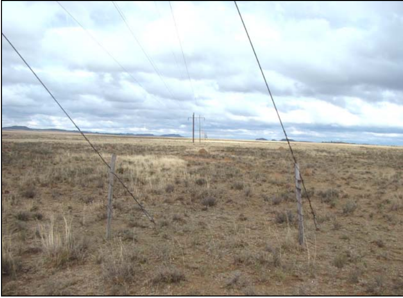
Fig.16 Pylon 101 on the Springfontein – Reddersburg line.
