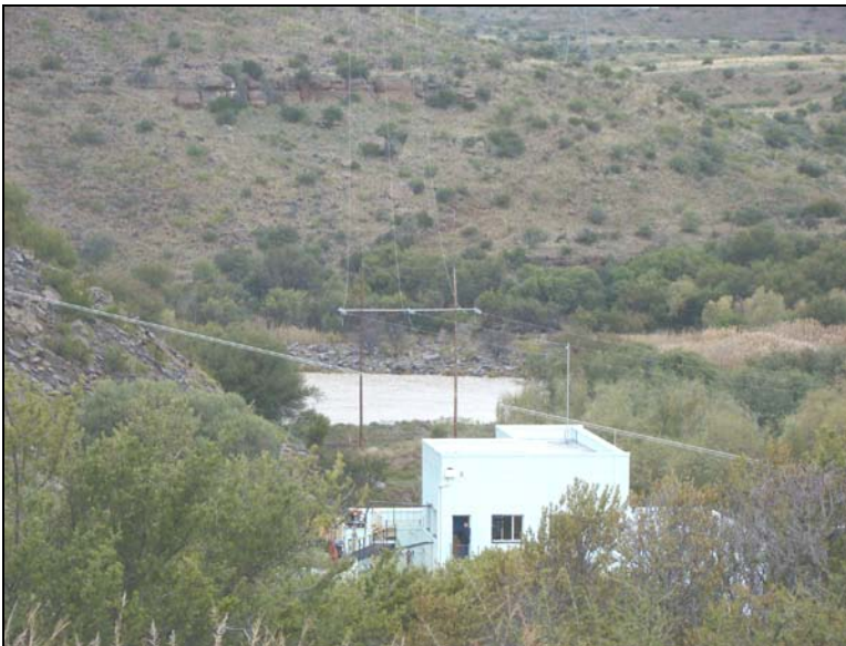
Fig.1 River crossing at Ruigtevallei Sub-station near Gariep Dam.
