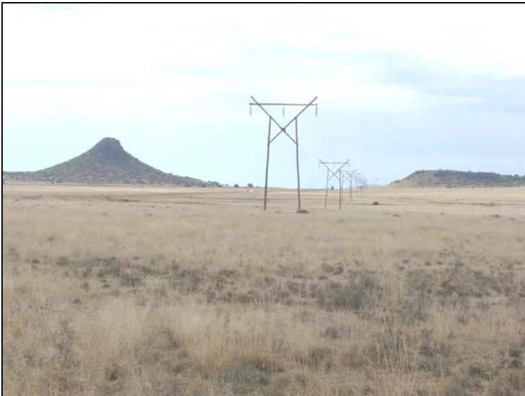
Fig.9 Pylon 222 on the Oranjekrag – Springfontein line.
