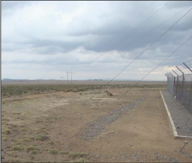
Fig.20 Edenburg Sub-station on the Edenburg – Reddersburg line.
