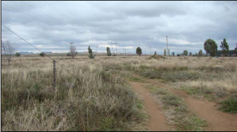
Fig.18 Pylon 148 on the Trompsburg – Reddersburg line.
