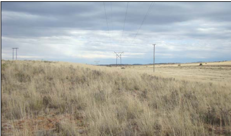
Fig.11 At Pylon 271 on the Oranjekrag – Springfontein line facing south.
