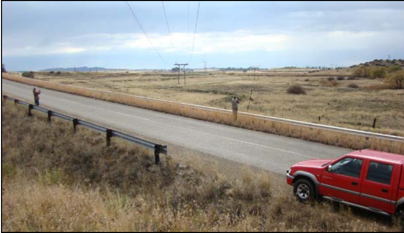
Fig.12 Pylon 271 on the Oranjekrag – Springfontein line facing east.
