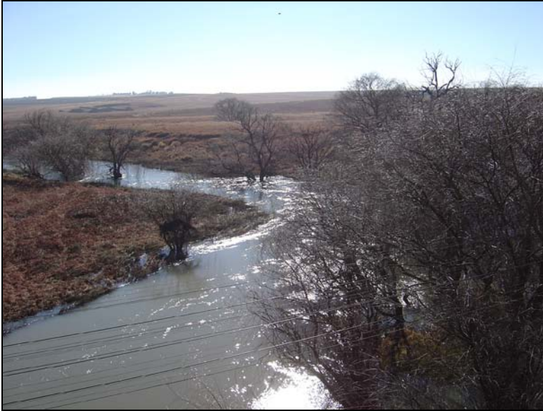
Fig.4 Liebenbergsvleispruit on the R57 between Reitz and Petrus Steyn.
