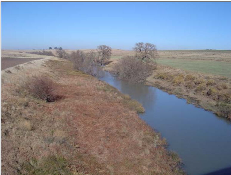
Fig.5 Liebenbergsvleispruit on the R57 between Reitz and Petrus Steyn.
