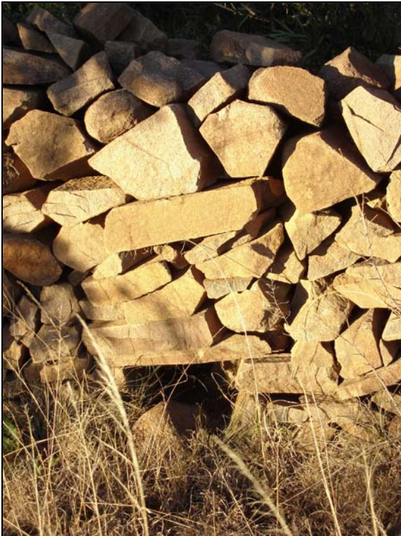
Fig.13 A drain-hole in one of the stone-walls at Katdoringfontein.
