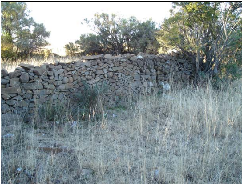
Fig.10 Outside of a well-preserved stone-wall at Katdoringfontein.
