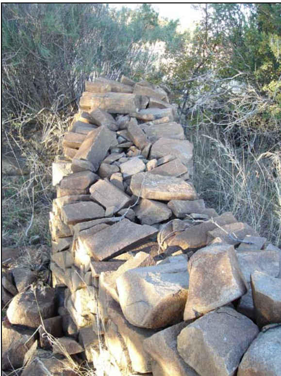
Fig.8 The structures represent the typical Later Iron Age walls of two separate parts on the outside with rubble in-fill.
