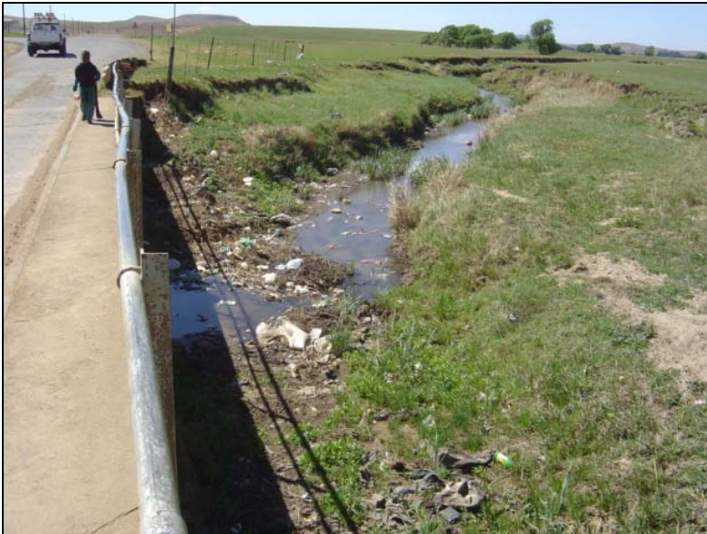
Fig.6 Bridge across the Pampoenspruit outside Memel.
