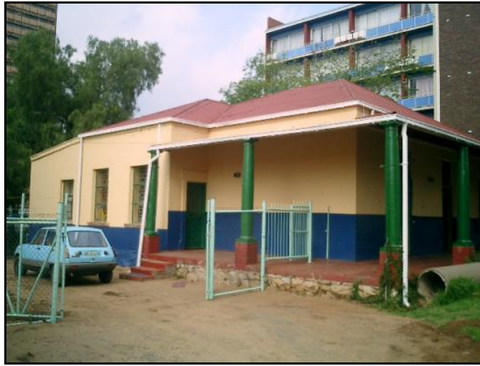
Figure 19: General view of 91 Charles Street with limited low impact recent alterations visible
