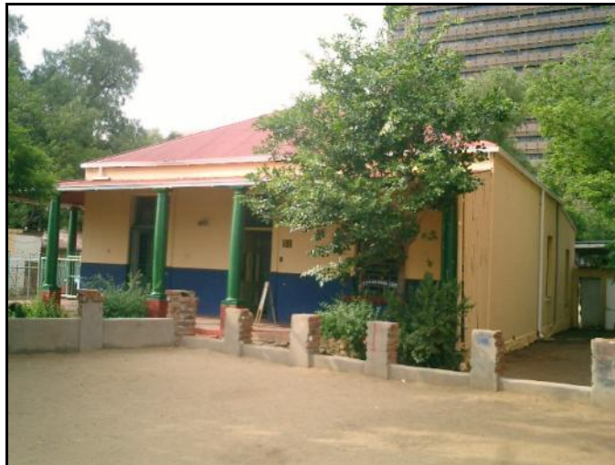
Figure 18: General view of 91 Charles Street
