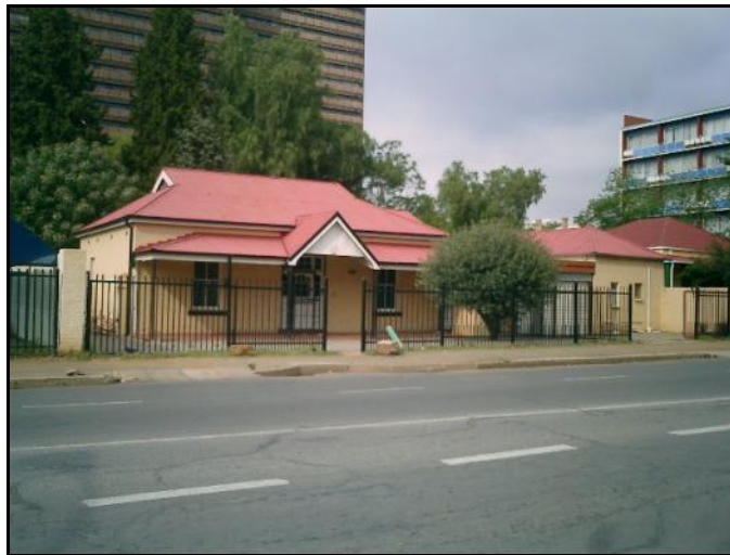
Figure 14: General view of 89 Charles Street
