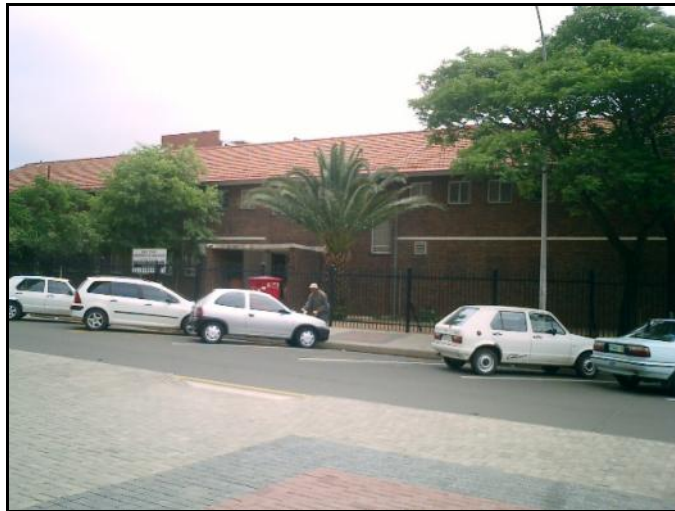
Figure 9: The contemporary Department of Education Building
