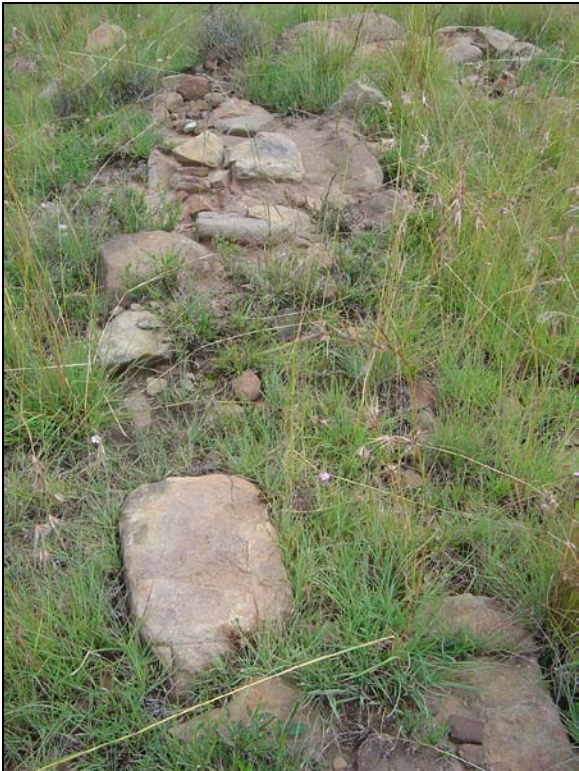
Fig.3 Foundation of a rectangular structure near borehole 3.
