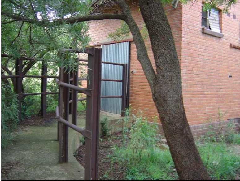
Fig.5 An old abattoir View along the proposed route of the pipeline.
