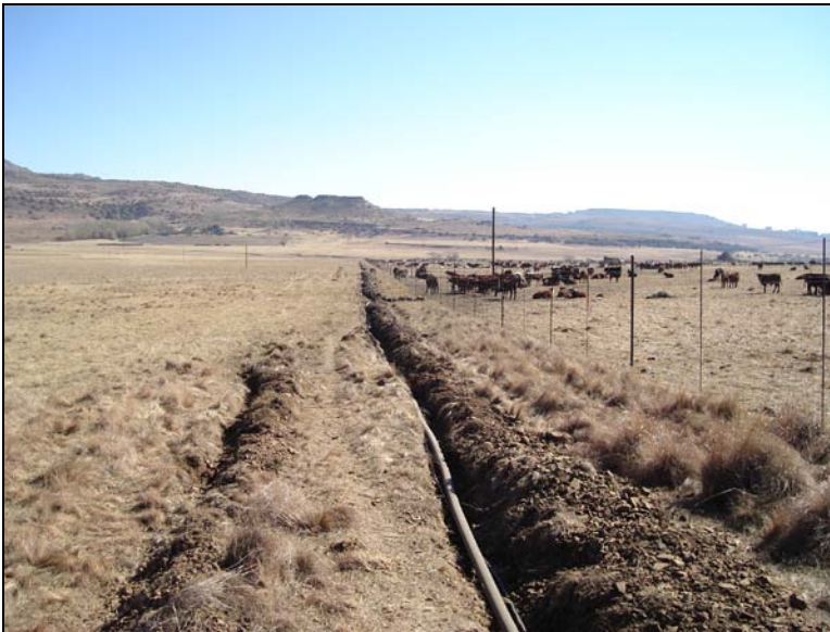
Fig.5 View from point 4 facing towards point 3.
