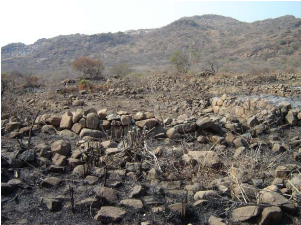
No. 2 Stonewalling after clearing of site
