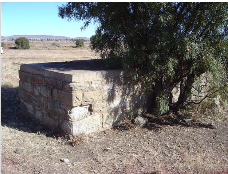
Fig.2 A stone and concrete structure, inscribed Thaba Nchu 33, is probably a tank stand near the bore hole T21118.
