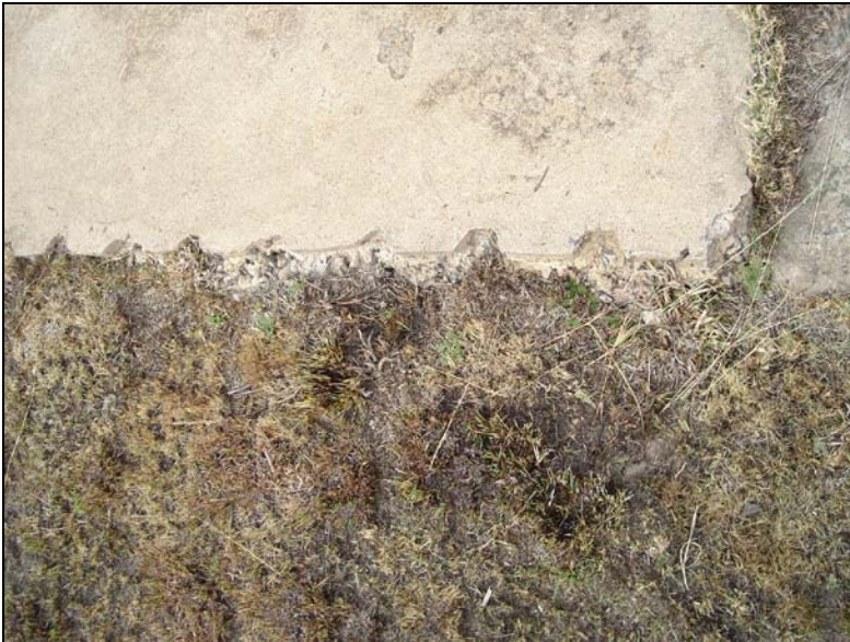
Fig.5 Impressions of an IBR type of corrugated iron in the concrete.
