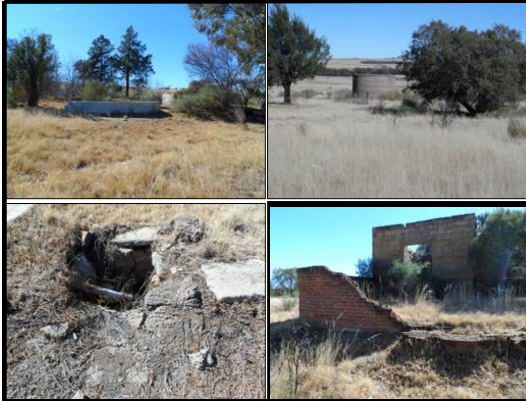
Figure 19 - Other site noticeable features such as the drainage system, reservoir, brick additions etc
