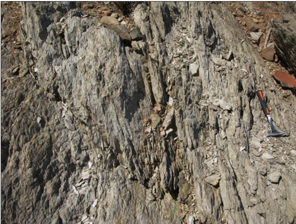
Fig. 5. Steeply-dipping, intensely-cleaved grey siltstones of the Klipbokkop Formation exposed in a road cutting about one kilometre NNW of the DR1392/3.3/L/10/A/R22 borrow pit site (Hammer = c. 30 cm).
