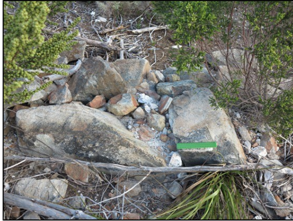
Figure 18: Detail of part of the east-west orientated wall showing the rubble infill. The ruler is about 15cm in length.
