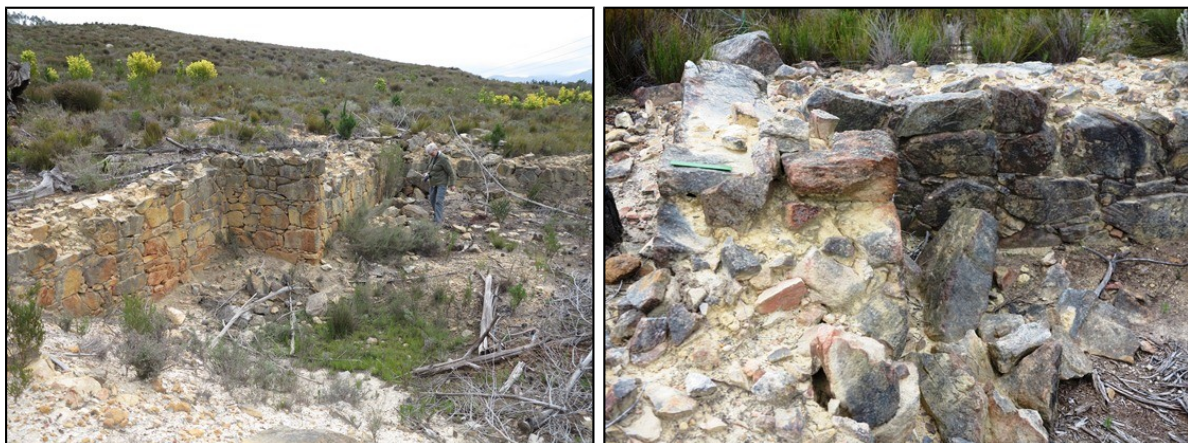
Figures 8 and 9: The stone ruin – view towards the west showing the sub-surface southern wall of the structure; detail of the northwest corner showing the rubble infill between the outer and inner stones. The ruler is about 15cm in length.
