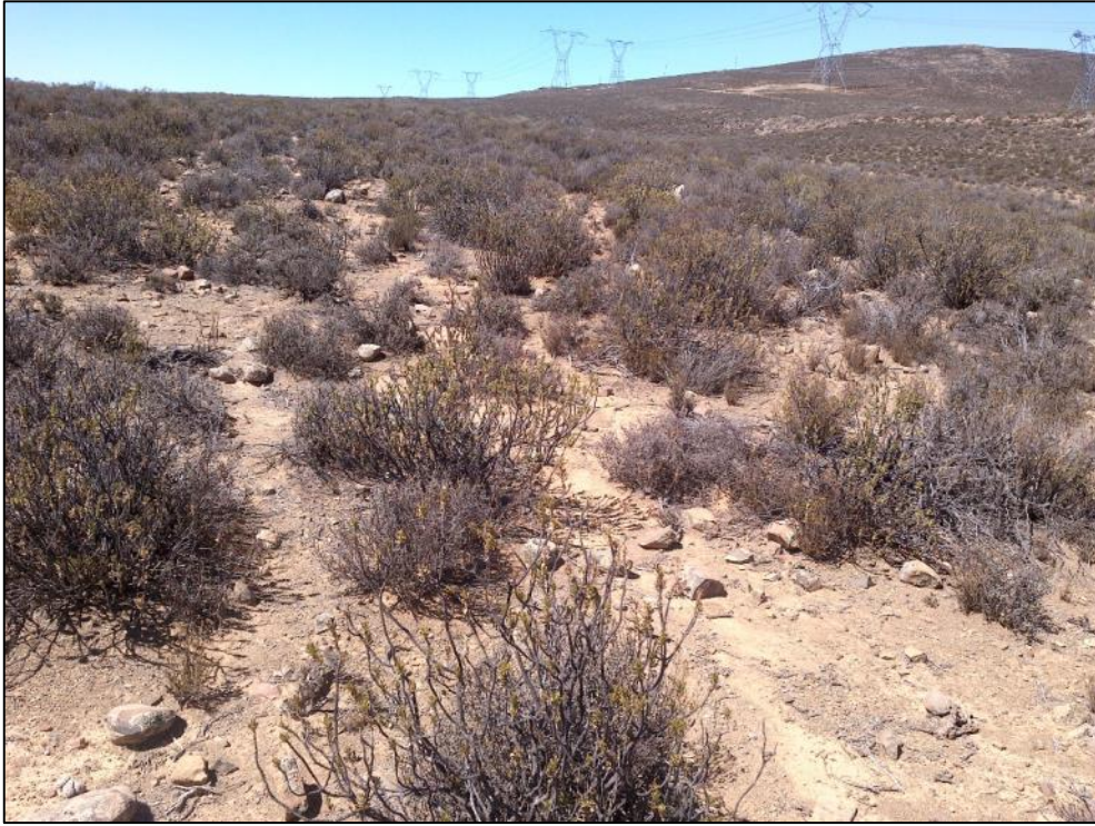
Figure 15: View of the area proposed for substation alternative SS2 facing south-east (Brandvalley 75).
