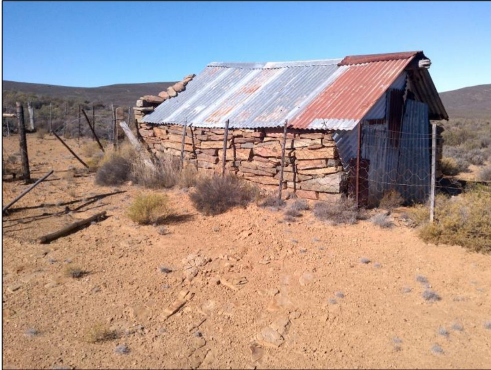
Figure 53: View of the modified stone walling cottage (BV_SW12) situated within the route proposed for the upgrade of the access roads.
