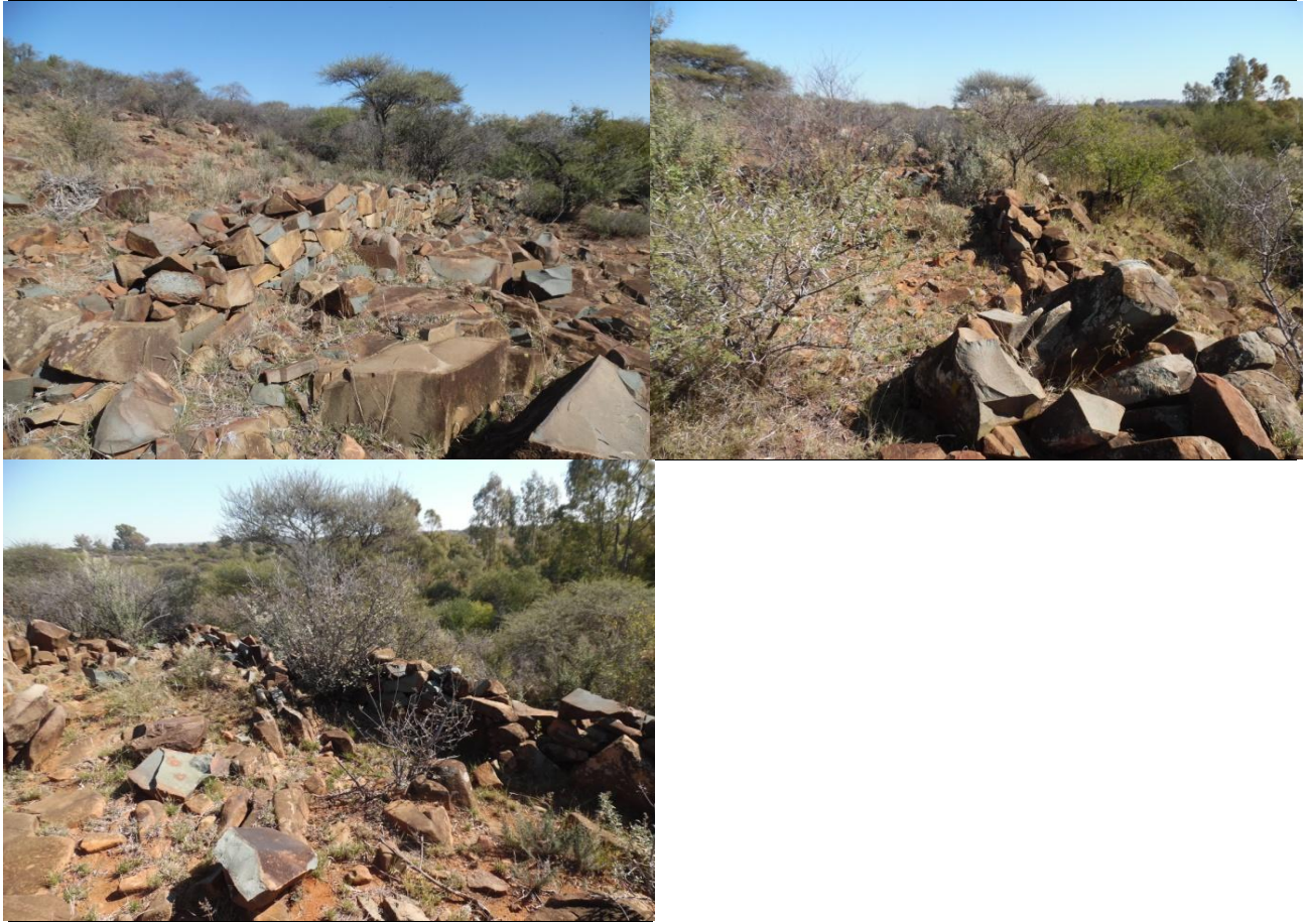
Figure 12- Stone wall terrace along the river banks (Warrington 1)
