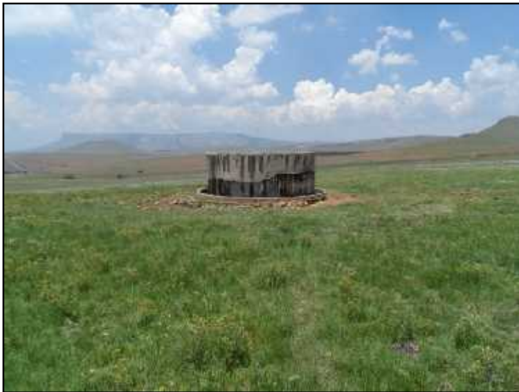
Figure 75 - Cement reservoir located in the middle of grazing fields
