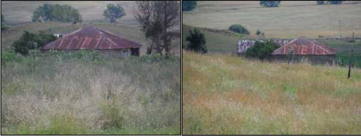
Figure 88 - Roofs of historic structures forming part of the historic farmstead
