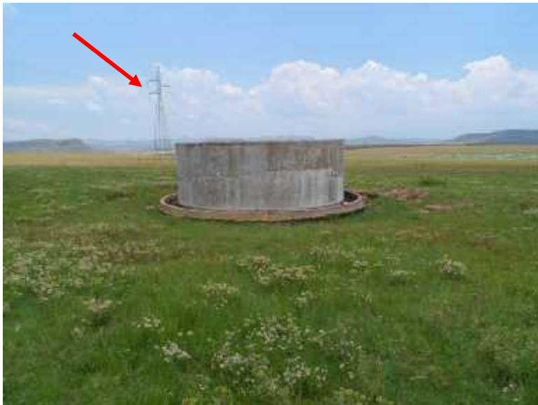
Figure 48- Reservoir in the middle of grazing fields. Note the existing power line in the background- red arrow.
