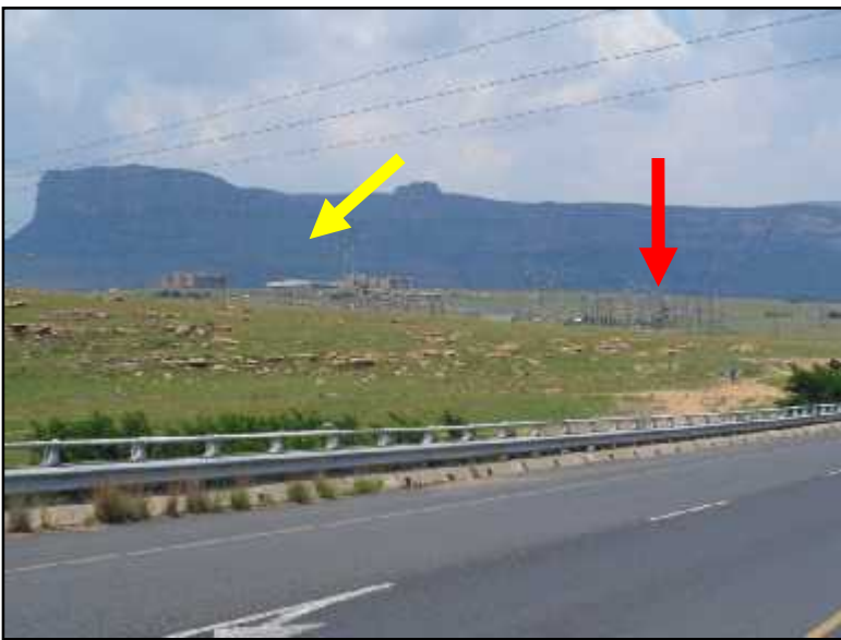
Figure 11- Witsieshoek Substation (red arrow) . Note University of the Free State Qwaqwa Campus in the background (yellow arrow)
