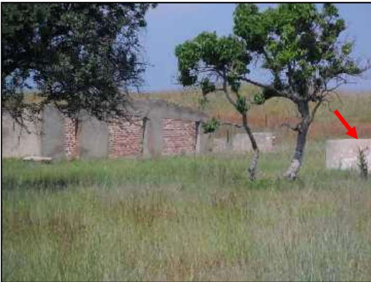
Figure 73 - Brick and cement shed. Note the 2 garage size doors and smaller door. Also note another smaller structure in front of the shed (red arrow)
