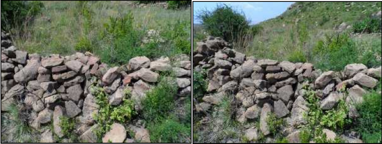
Figure 97 - Picture showing one of the kraals well preserved walls. Note the subdivisions inside the kraal.
