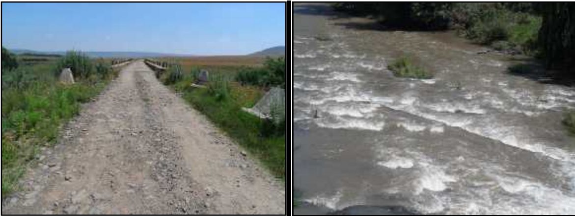
Figure 6- Wilge River pictures. One showing a bridge (left picture) and the other (right picture) the main river channel south-west of where Corridor 2 joins Corridor 1.
