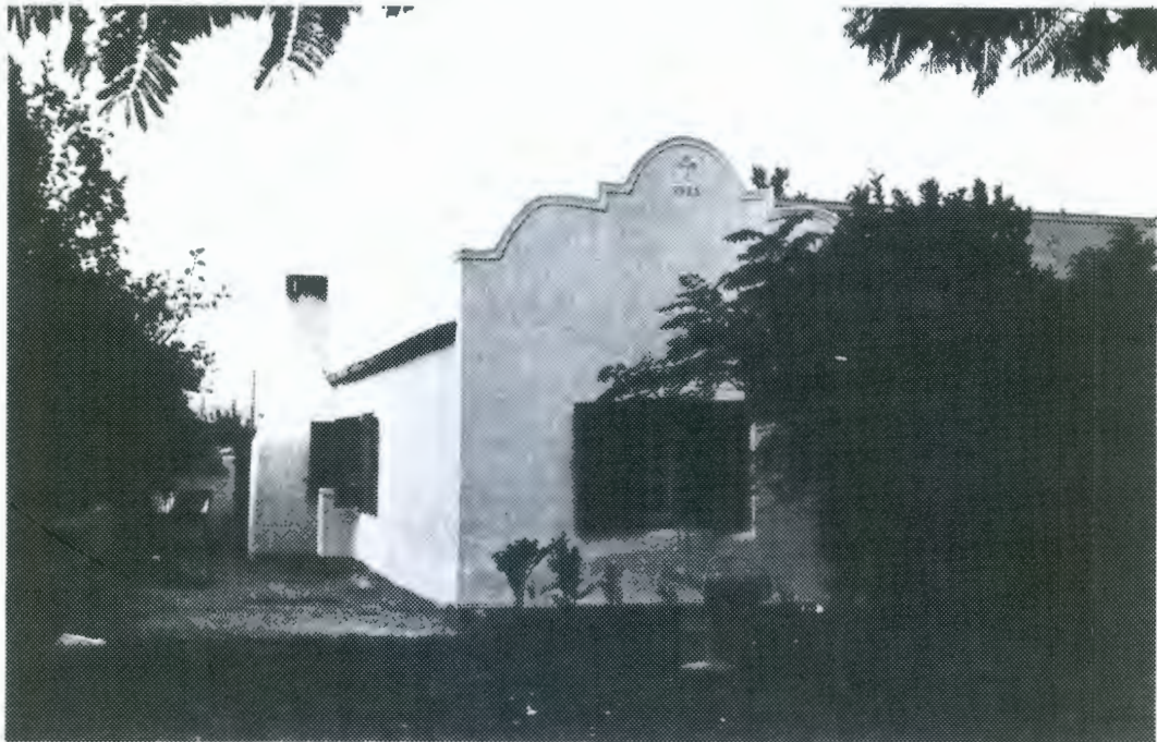
House with corrugated iron roof and projecting Cape Dutch revival gable, dated 1935. Verandah on plastered columns. 6 x 6 sashes with louvred shutters.
