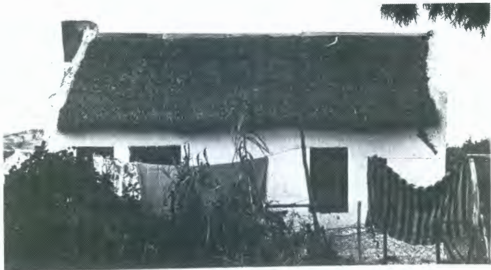
Vernacular cottage with reed thatch, triangular end gables and external chimney. 6-pane casements.
