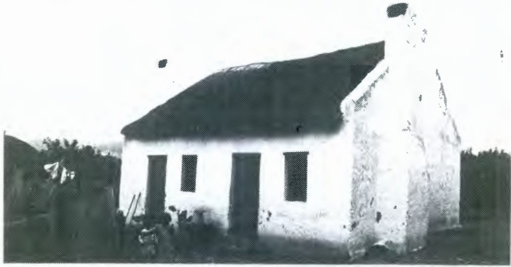
Vernacular cottage with reed thatch, straight end gables and two external chimneys. 6-pane casements, stable doors.
