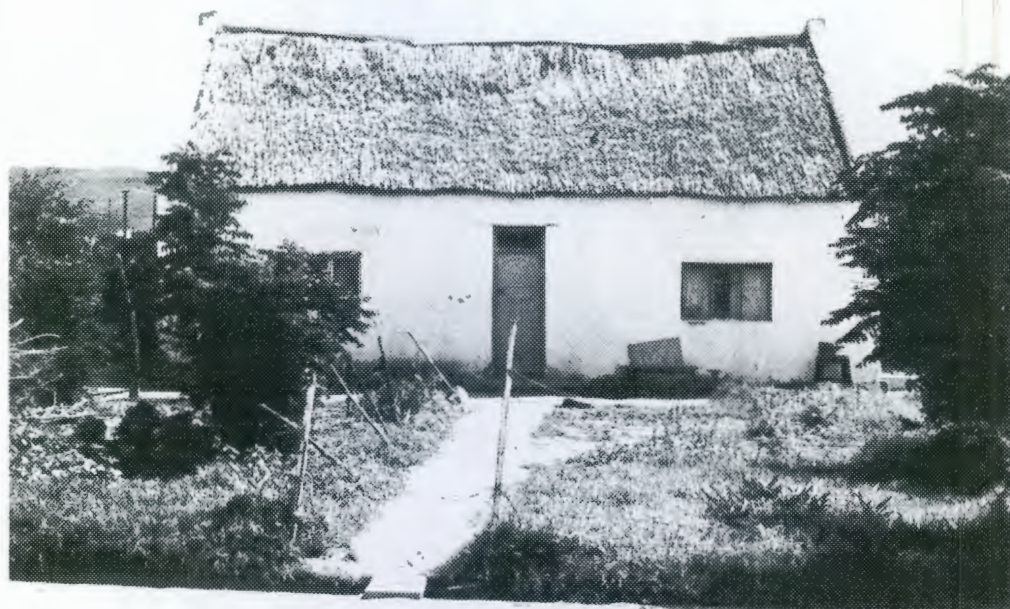
Vernacular cottage with reed thatch, straight end gables and external chimney. Steel windows, 3-panel Edwardian door with 2-pane fanlight.
