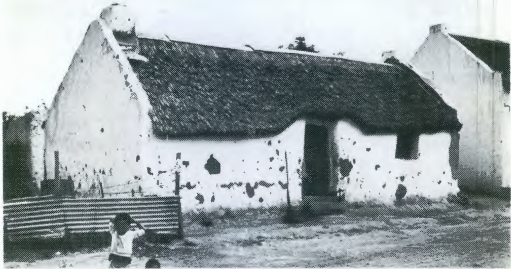
Vernacular cottage with reed thatch, straight end gables and internal chimney. Low hood over stable door. Small casement.
