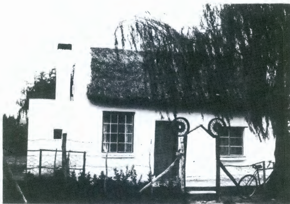
Vernacular cottage with reed thatch, straight end gables and external chimney with small window. 8 x 8 casement and steel window; stable door. Extension at rear with monopitch roof and steel windows.
