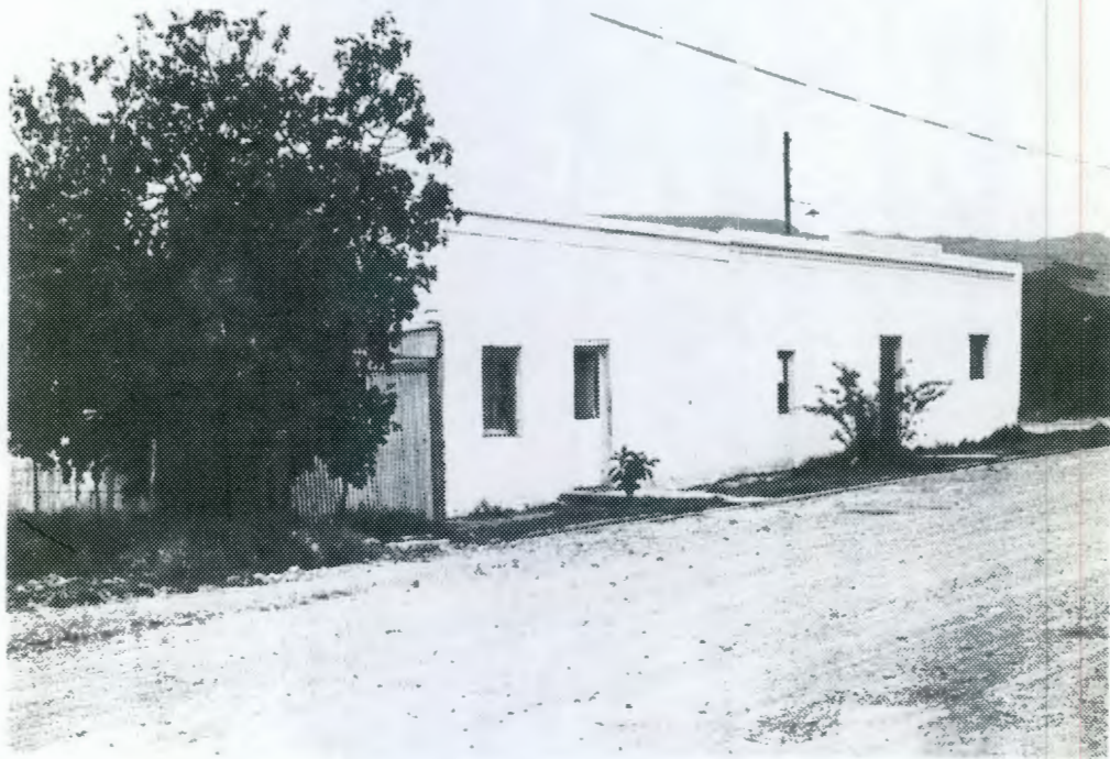
Semi-detached cottages with stepped-up parapet and cornice. 2 x 2 and 1 x 1 sashes and 6-pane casement. Stable doors.
