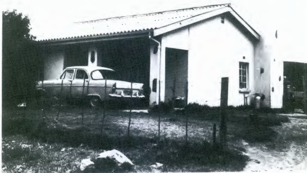
Modern house with asbestos saddle roof with covered end gables, recessed porch and steel windows. External chimney with inset slate.
