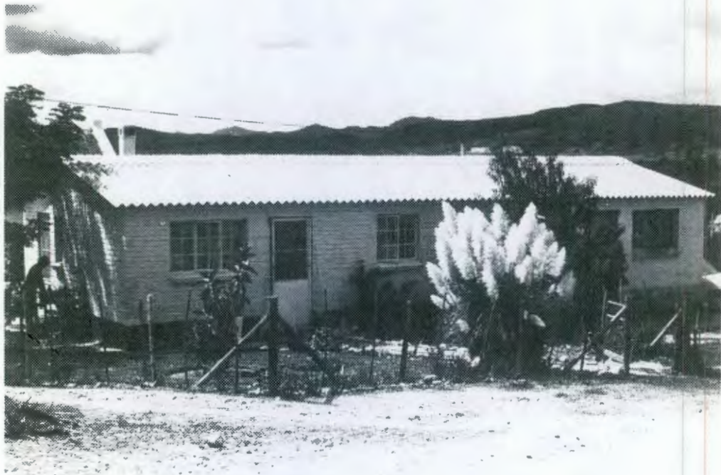
Housing scheme with 4 semi-detached houses on erf 371 and 8 on erf 370. Houses are painted facebrick with asbestos saddle roofs, steel 6-pane combination casements and modern doors.
