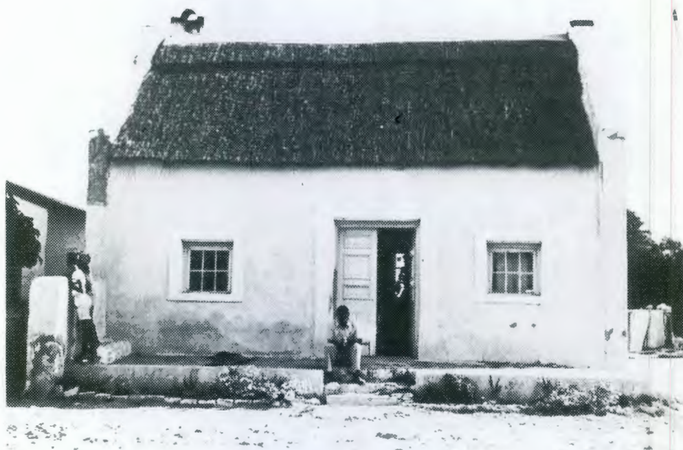
Vernacular cottage with thatched roof and straight end gables. 4 x 4 panel doors with lowest mouldings missing. 6-pane casements. Plaster surrounds to openings. Stone stoep with one end wall with low seat.
