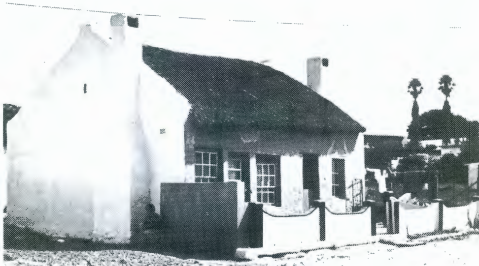
Vernacular cottage with reed thatch, straight end gables and external chimneys. 6 x 6 sashes, glazed and stable doors. Wall with posts and dipped panels.
