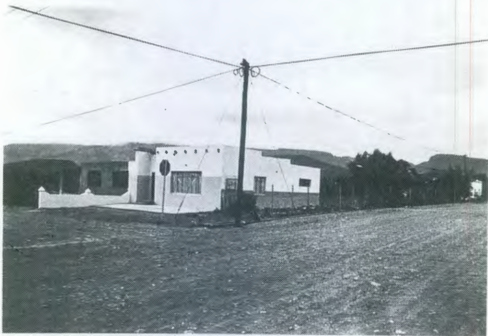
BUSY CORNER CAFE House with parapeted roof with exposed rafter-ends. Modern windows and door. Wall with capped posts.
