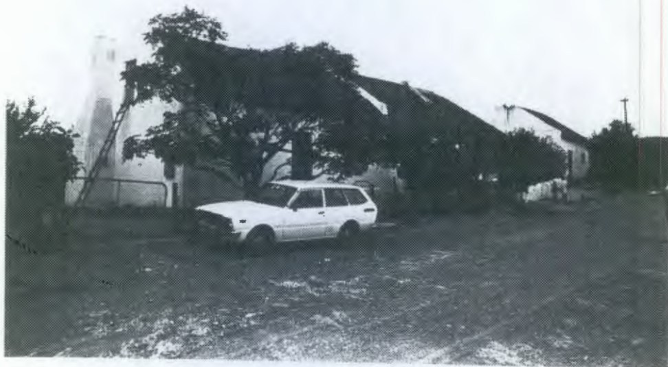
Row of three attached cottages with thatched roofs. 'A' has a straight end gables, loft door with ladder and external chimney with small window. Steel windows, door with 4-pane casement. 'B' has a 6 x 6 sash. 'C' has a hipped, thatched roof, steel window and door with geometric glazing.
