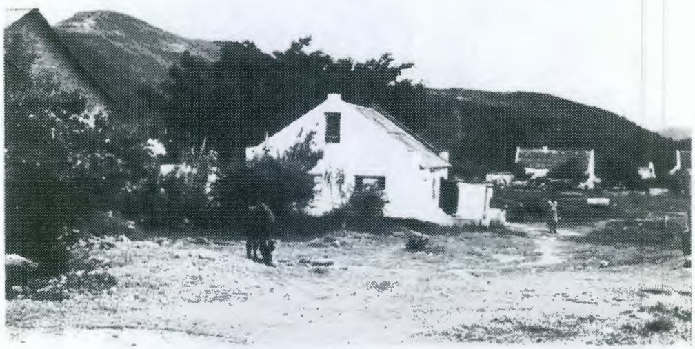
Cottage with corrugated iron roof, straight end gables and 6-pane casement to loft.
