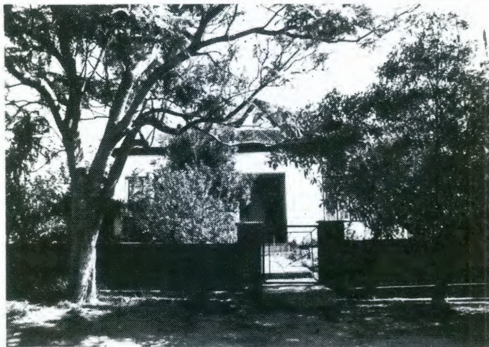
House with hipped, thatched roof with triangular, louvred dormer above front door. Recessed entry with 3-panel door with side- and fanlights. Recessed verandah enclosed with steel windows. Composite 6-pane casements with 4-pane fanlights.
