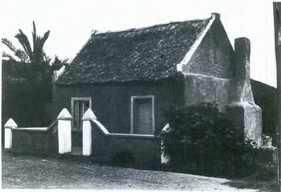
Vernacular cottage with reed thatch, straight end gables and external chimney. Steel casement and stable door with plaster surrounds. Plastered wall with capped posts.
