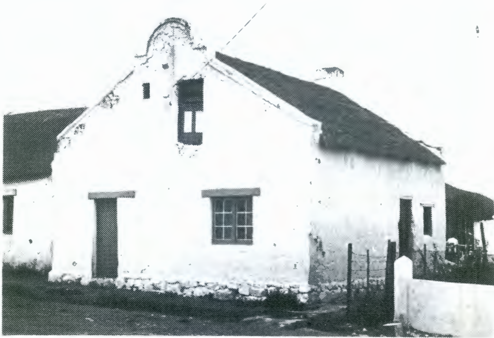
Thatched cottage with round-topped end gable and off-centre loft door. 6 x 6 and 4-pane casements and doors, all with exposed wooden lintols.
