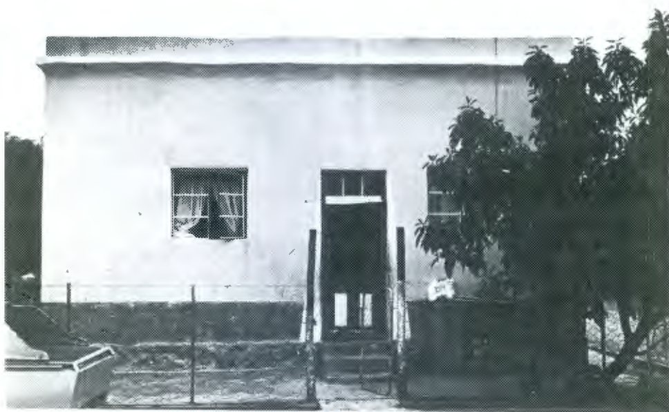
Vernacular cottage with parapet and cornice. Steel windows. 2 x 2 panelled stable door with 3-pane fanlight.
