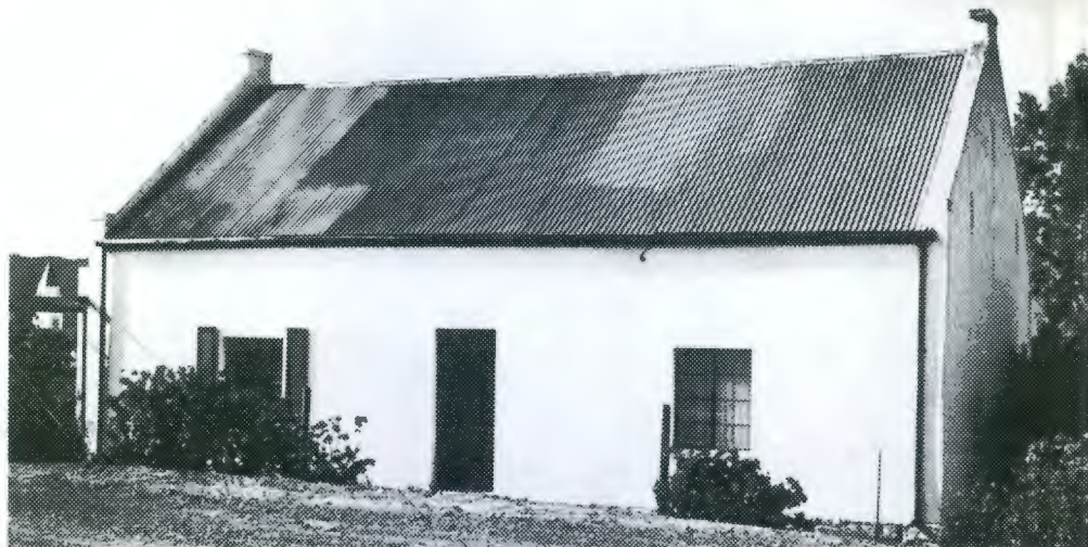
Cottage with corrugated iron roof and straight end gables. Steel windows, modern glazed door.
