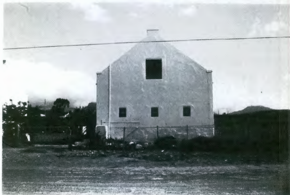
Cottage with thatched roof and straight end gables. End gable facing street has loft window divided into four, with 4 panes per quarter, and three small 4-pane windows. The long facade has cast iron vents under the eaves. 6 x 6 sashes; 4-panel door and corrugated iron garage doors. Pergola on capped, plastered columns, with wooden cross-braced balustrade.
