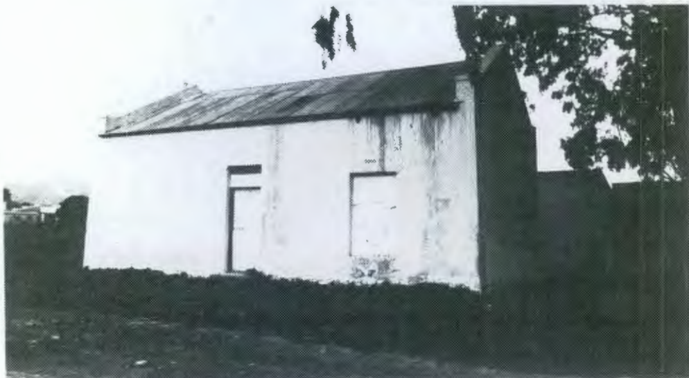
Vernacular cottage with corrugated iron roof triangular end gables and external hearth. Stable door with fanlight (boarded up) and boarded up window.
