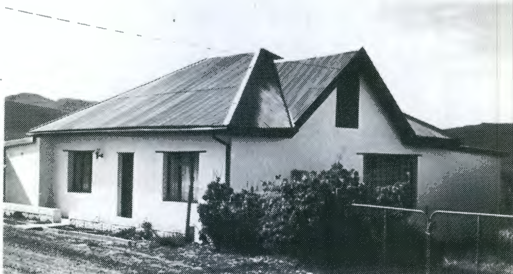
House with hipped iron roof with a covered gable with loft door on the side. Steel windows, modern door.
