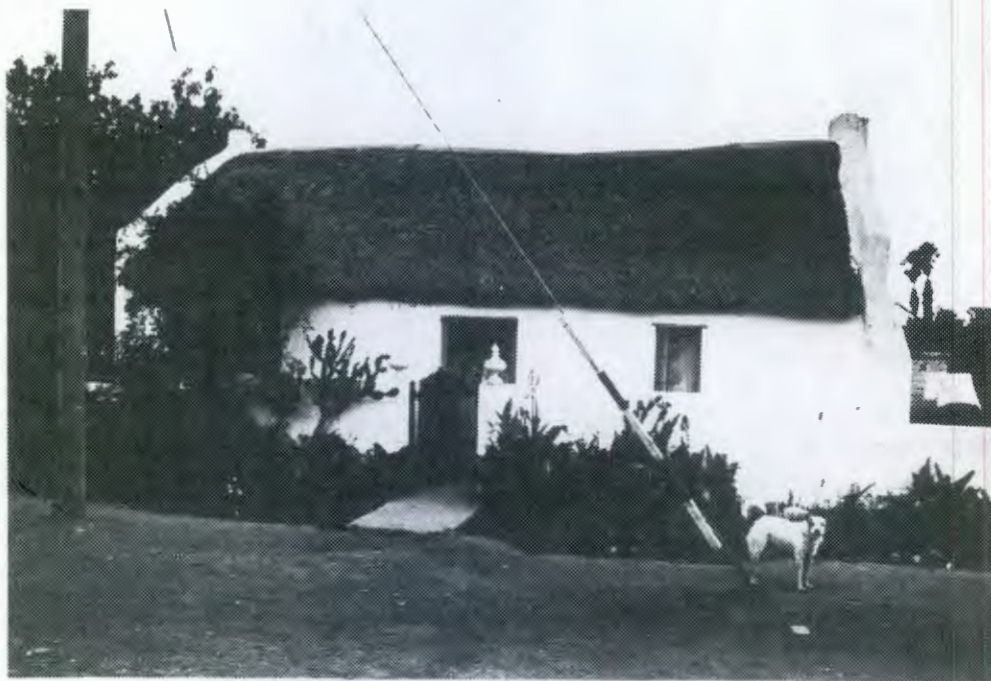
Vernacular cottage with reed thatch and straight end gables with external chimney. Stable door, steel casements.
