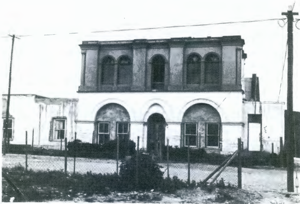
3-bay double storey building with parapet. Upper floor has 4-pane windows with sunrise fanlights, paired on the outer bays and separated by pilasters. Corresponding blind niches on side elevation. Columns inset at the corners. Ground floor has large arches over paired 2 x 2 sashes. Central arch has trefoil arch inset, over double doors with arched upper panels and fanlight (missing). Lower part of ground floor is coursed stonework. Right-side has projecting room with parapet, 2 x 2 sash and stable door with 4-pane fanlight. Left side has parapeted, single storey extension with 2 x 2 sashes.
