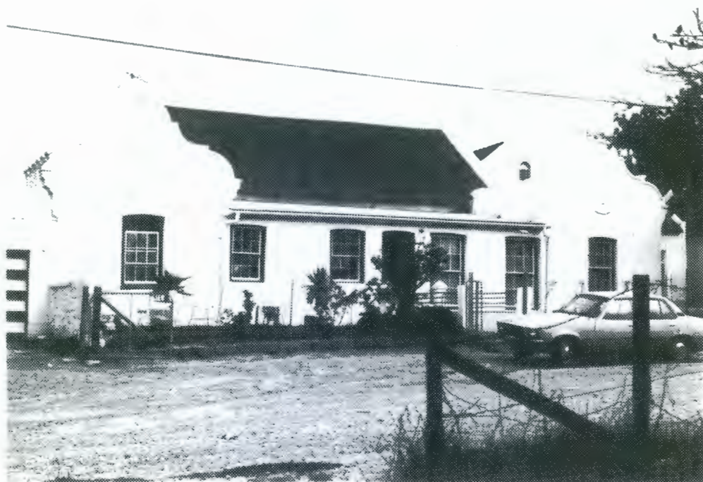
Vernacular cottage with thatched roof and straight end gables. Extension in front with two Cape Dutch revival gables with large plaster medallions and castellated parapet behind. Corrugated iron roof between. 6 x 6 sashes with quoins.
