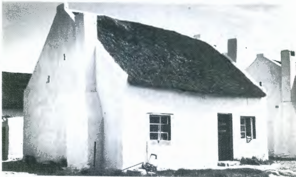
Vernacular cottage with thatched roof, straight end gables and external chimneys. Steel windows with painted quoins. Glazed door.
