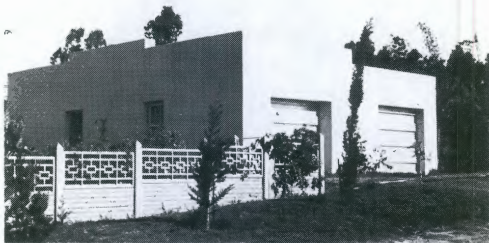
Double garage with stepped-up parapet, 6 x 6 sash and tip-up garage doors.
