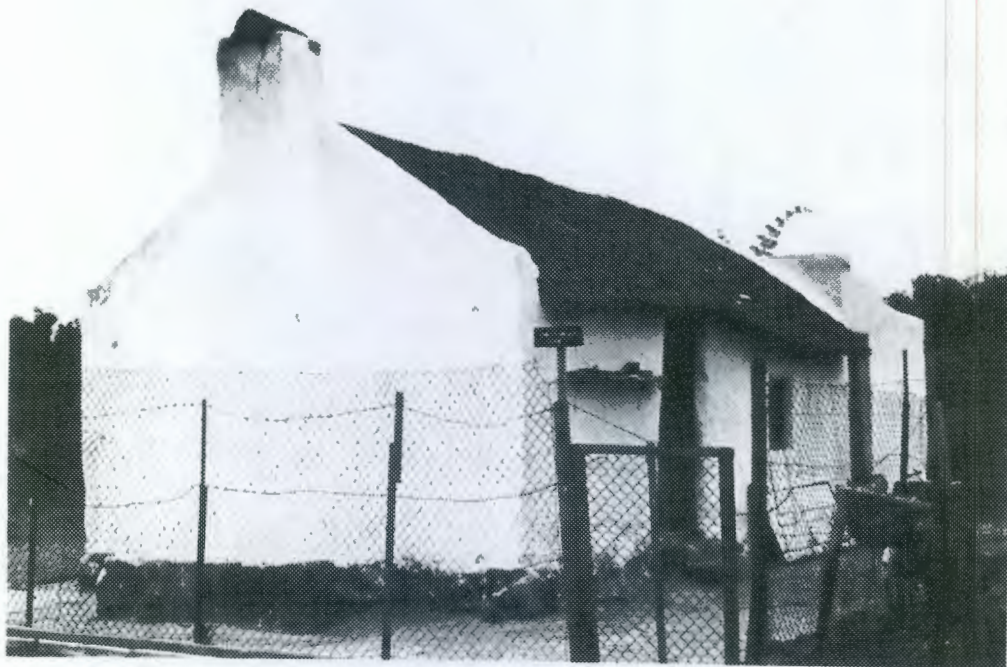
Vernacular cottage with reed thatch, triangular end gables and external chimney. Stable door and small casement. Small extension with stepped-up parapet.
