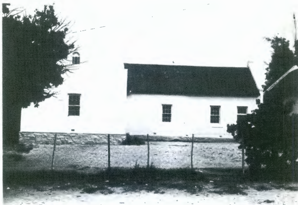
L-shaped, thatched building with one straight end gable and one Cape Dutch revival gable, dated 1930, with arched, louvred vent. 6 x 6 sashes with plaster surrounds. Panelled double door with fanlight.
