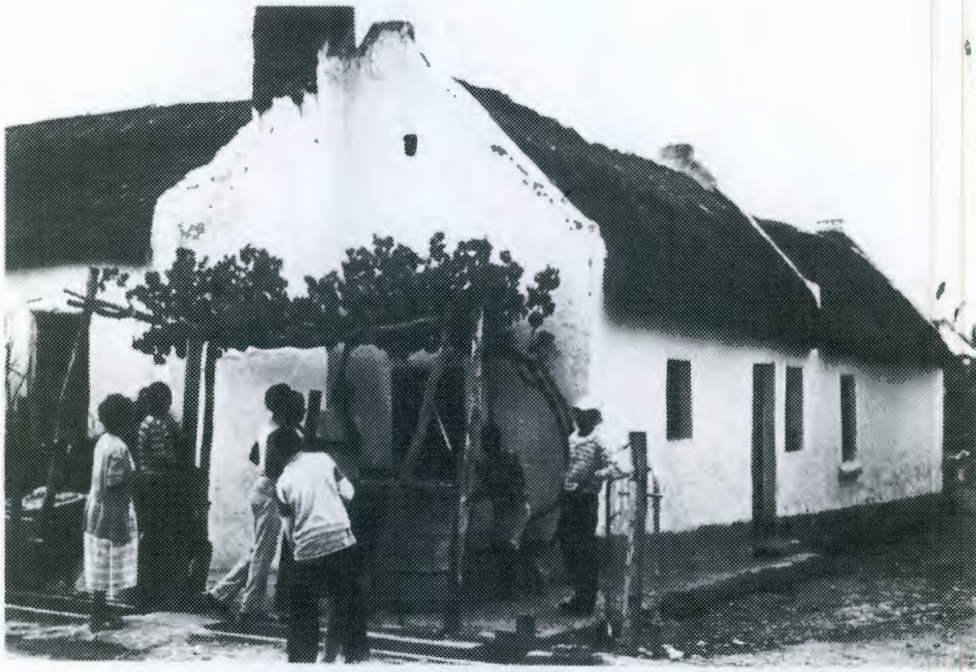
Vernacular cottage with reed thatch, straight end gables and external chimney. Stable doors, small casements.
