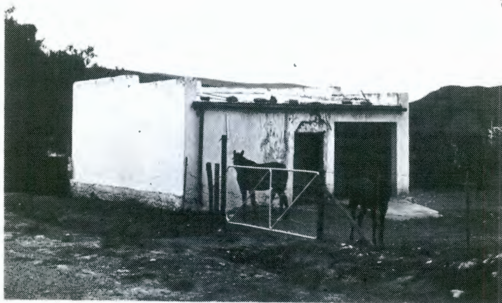
Parapeted outbuilding with iron roof, stable door and modern garage door.
