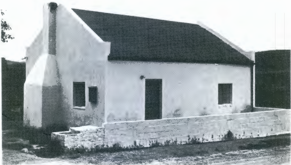
Modernized vernacular cottage with corrugated iron roof, triangular end gables and external chimney. Steel windows, stable door.
