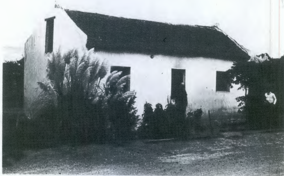
Vernacular cottage with reed thatch, straight end gables and loft door. Small casements.
