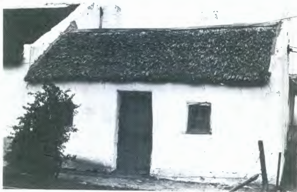
The one on the right is smaller, with straight end gable and reed thatch. Small 4-pane casements, stable door.
