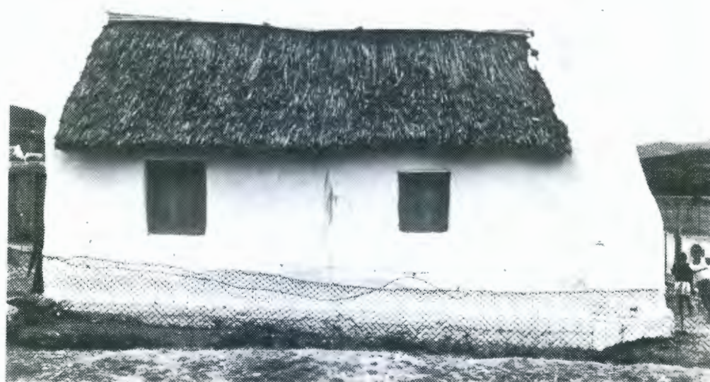
Vernacular cottage with reed thatch, triangular end gables and external chimney. 4-pane and single-pane casements.
