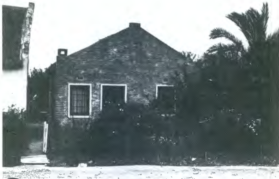
Vernacular cottage with thatched roof and straight end gable facing the street. Gable is bagged brick, with plaster surrounds to 12-pane windows and 4-pane door.
