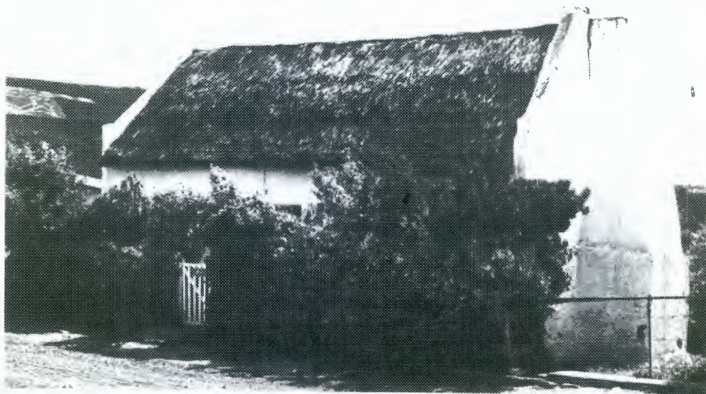
Vernacular cottage with reed thatch, straight end gables and external chimney. Steel windows.
