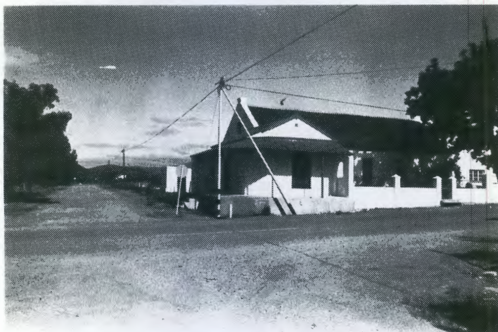
Vernacular cottage with fancy thatching, straight end gables and loft door. 6 x 6 sashes, door with fanlight. Victorian addition on corner, at right angles to cottage. Corrugated iron saddle roof with finial. Splay at corner verandah on pipe columns, with wooden fretwork. 2 x 2 sash with louvred shutters, door with window panes. Plastered garden wall with posts and railing.
