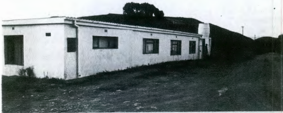
Modern house with monopitch IBR roof and wooden fixed-pane/casement windows.
