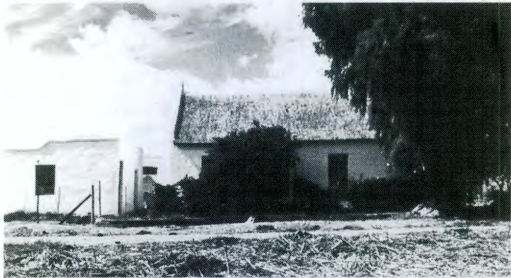
Vernacular cottage with thatched roof, straight end gables and external chimney with rounded top. 12-pane casements. Stable door.
