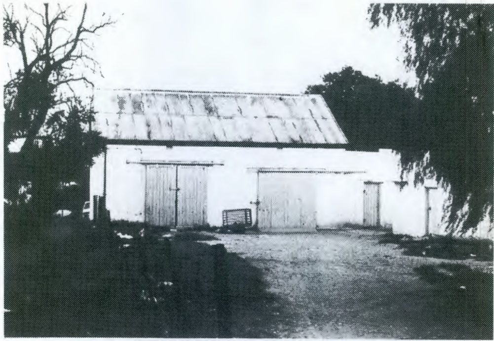
Outbuilding with corrugated iron saddle roof. Corrugated iron and wooden sliding doors.
