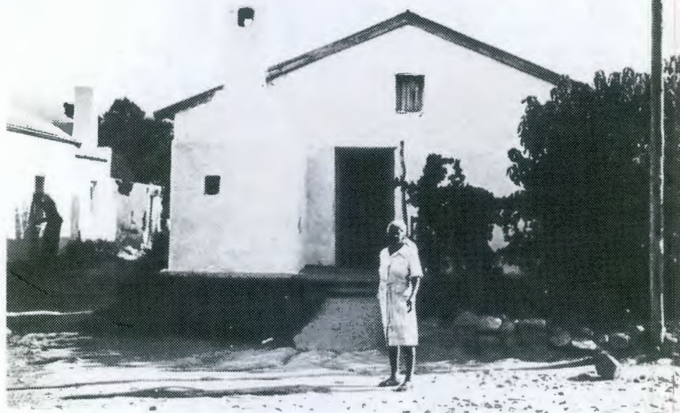
House with low-pitch corrugated iron saddle roof with covered end gable facing street. Loft window (boarded up), plain door and external chimney on gable end.
