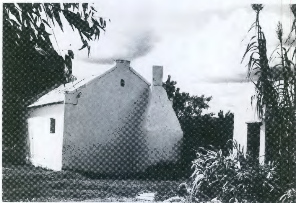
Vernacular cottage with corrugated iron roof, straight end gables and external chimney. Small casement windows.
