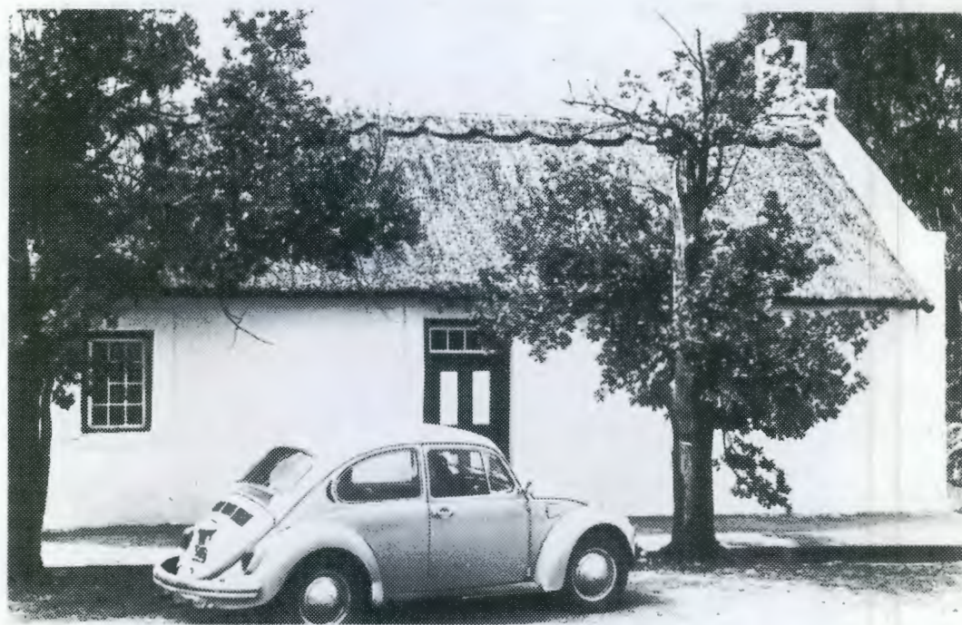
Vernacular cottage with fancy thatching, straight end gables and internal chimney. 12-pane casements and 4-pane door with 4-pane fanlight. Extension with lower thatched roof and straight end gable.
