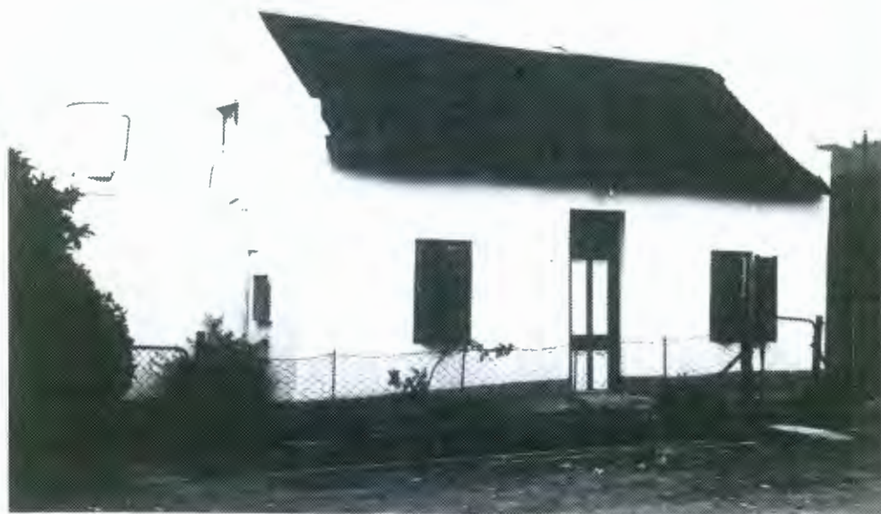
Vernacular cottage with thatched roof, straight end gables and loft door. 6 X 6 sashes with louvred shutters, 4-panel door with fanlight. Extension with fancy stepped-up parapet.
