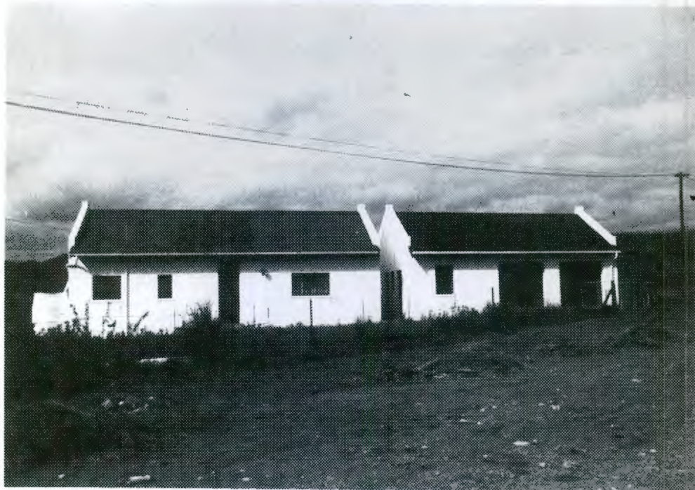
Cottage and adjacent garage with straight end gables and corrugated iron saddle roofs. Composite 6-pane wooden casement windows. Narrow door. Garage has two garage doors and 6 x 6 sash.
