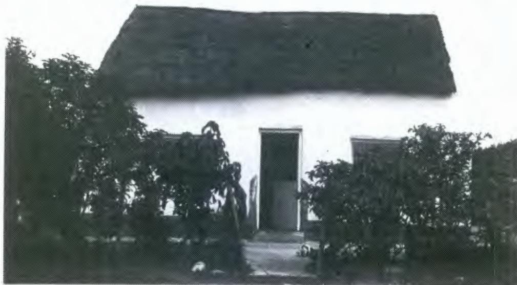
Vernacular cottage with thatched roof and straight end gables. Stable door, wooden small-pane casements.
