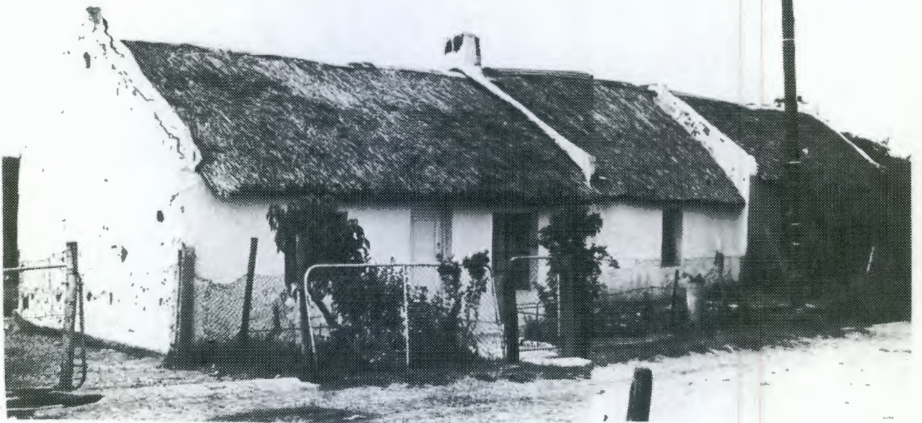
Vernacular cottage in three sections, with reed thatch and straight end gables. 6 x 6 sash, 6-pane casement and steel windows.
