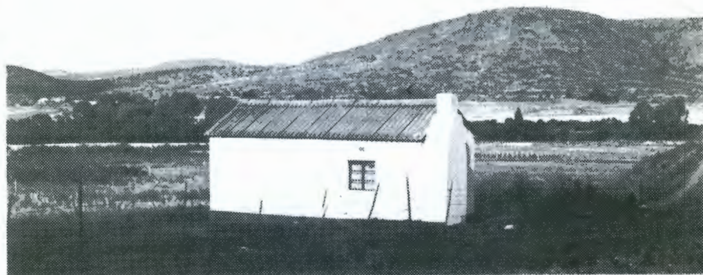
Small cottage with asbestos saddle roof, external chimney and steel windows.
