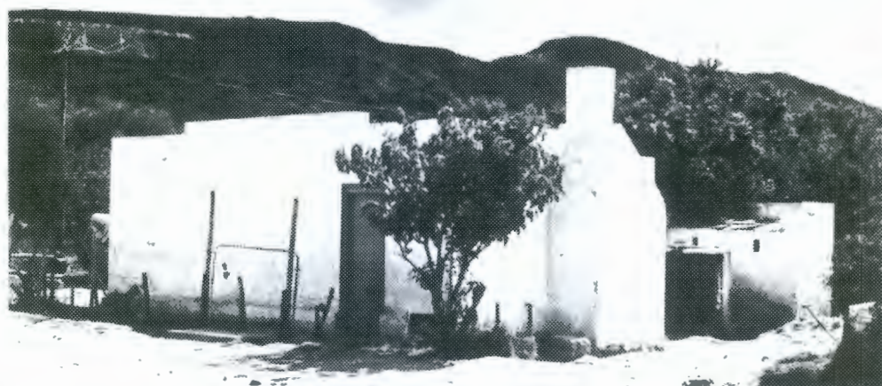
Vernacular cottage with stepped-up parapet and external chimney. Stable door. No windows on street side.
