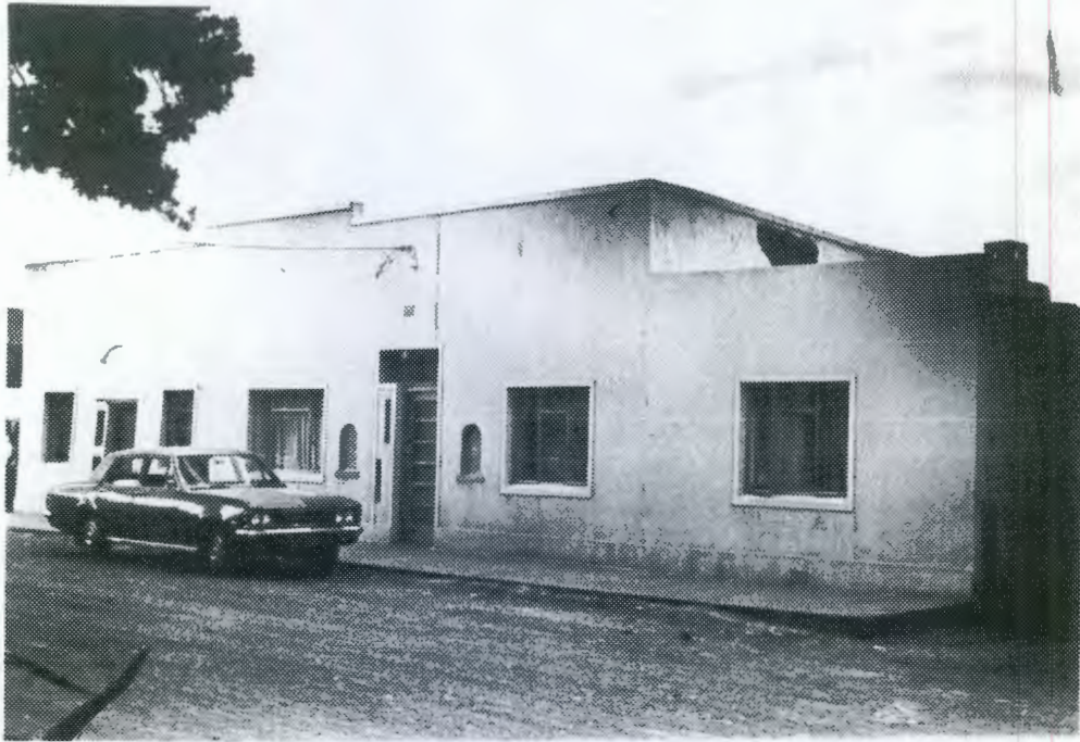
Building with stepped-up parapet. Steel windows. Stable door, modern glazed door with wider 4-pane fanlight. Adjacent outbuilding with corrugated iron roof, straight end gables.
