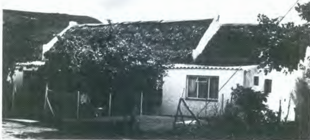
Vernacular cottage with reed thatch and straight end gables. Thatched room added longitudinally. Rooms built on in front with asbestos roof and steel windows.
