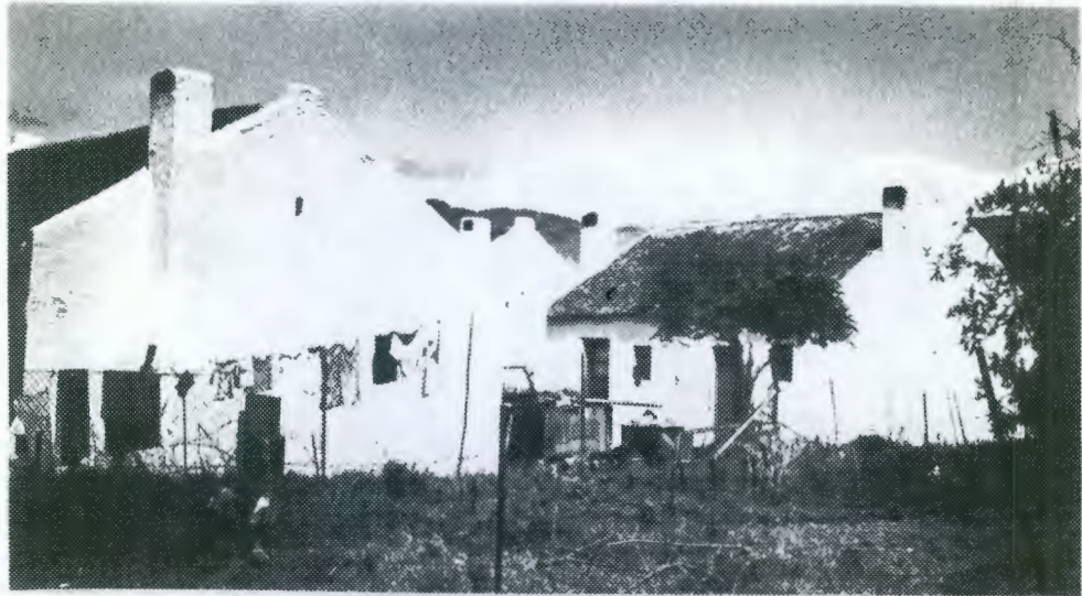
Vernacular cottage with reed thatch, straight end gables and external chimneys. Glazed and stable doors. Small casements.
