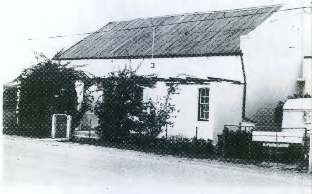
Cottage with corrugated iron roof, straight end gables, external chimney and loft door with staircase. 6 x 6 sashes. Pergola on plastered columns.
