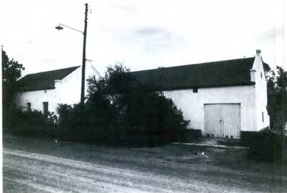
Adjacent garage with corrugated iron roof and straight end gables with diamond windows. Wooden double doors. Stone plinth.
