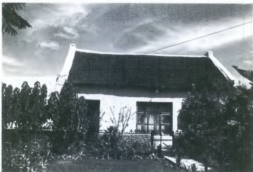
Vernacular cottage with thatched roof, straight end gables and parapeted extension on left. Large, modern wooden window. Low boundary wall with cast iron cresting.
