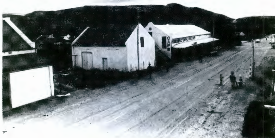
Outbuilding with corrugated iron saddle roof with traingular gable end towards street; loft door.
