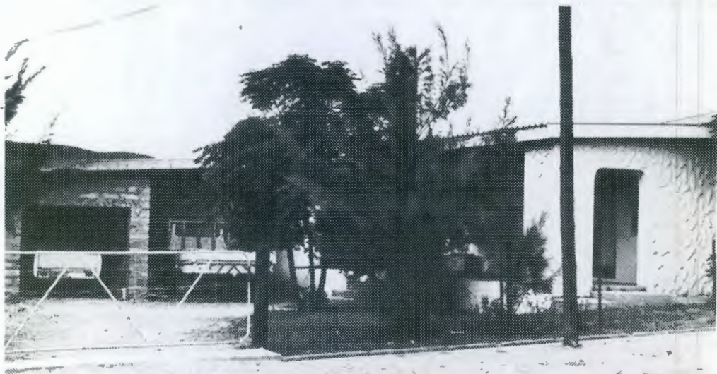
Modern house with monopitch IBR roof, textured plaster and recessed porch. Attached garages roughly built of concrete blocks.
