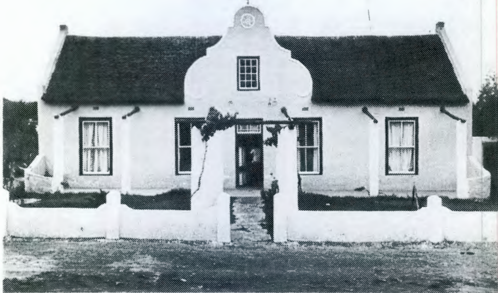
House with thatched roof and straight end gables, with holbol front gable and 12-pane loft window. 2 x 2 sashes. Panelled door with geometric fan=light. Steep with curved end walls and gumpole pergola on plaster columns. Pergola over path. Low plastered wall with posts.
