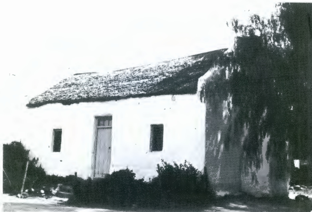
Vernacular cottage with reed thatch, straight end gables and external chimney. Loft door. 6-pane casements. Door with 3-pane fanlight.
