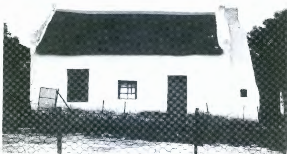
Vernacular cottage with reed thatch, straight end gables and external chimney with small window. Stable door, 6 x 6 sash and small steel casement.
