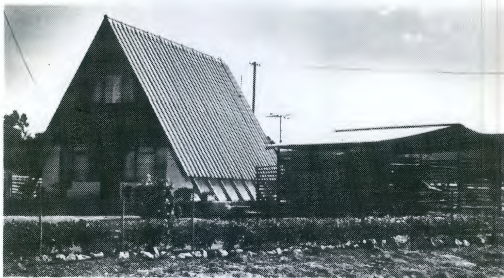
A-frame house with wooden cladding to upper floor. Steel windows, stable door. Carport with low-pitch corrugated iron saddle roof.
