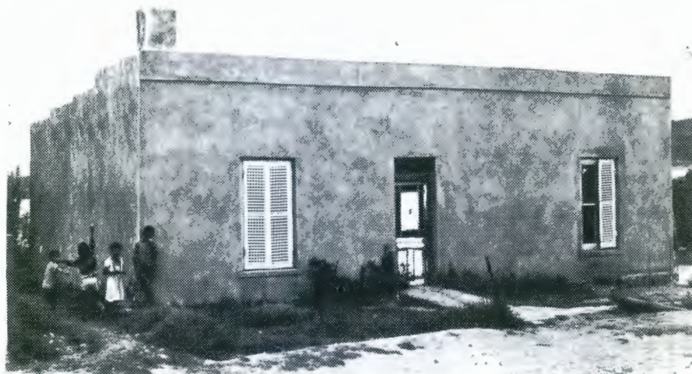
Vernacular cottage with parapet. 2 x 2 sashes with louvred shutters. Door with geometric glazing and 3-pane fanlight.
