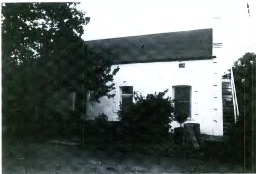
House with corrugated iron roof and straight end gables with plaster moulding. Quoins to corners, windows and doors. 2 x 2 sashes. Glazed Victorian door with fanlight and coloured glass. End gable has loft door and wooden stair.
