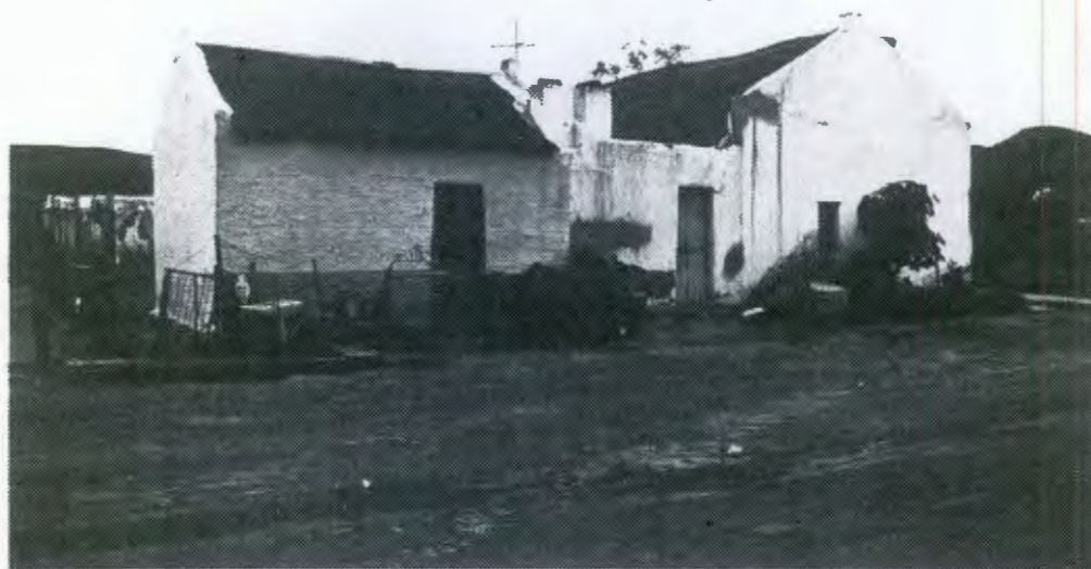
Two vernacular cottages with thatch and straight end gables, with parapeted connection. Stable doors, small casement.
