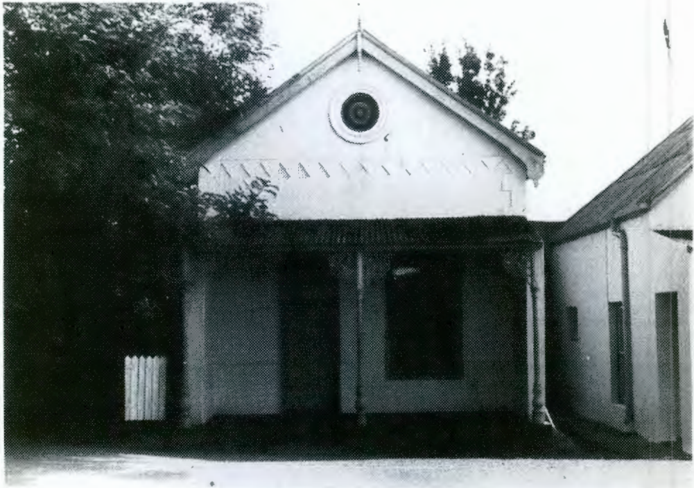
Victorian cottage with covered gable facing street. Tall finial and barge boards with pendants. Round cast iron vent. Plaster decoration includes moulding around vent, chevron pattern above verandah and quoins to corners and door (now partially obscured). Verandah with cast iron columns and brackets and side walls. 3-panel door with fanlight. 2 x 2 sash with internal shutters.
