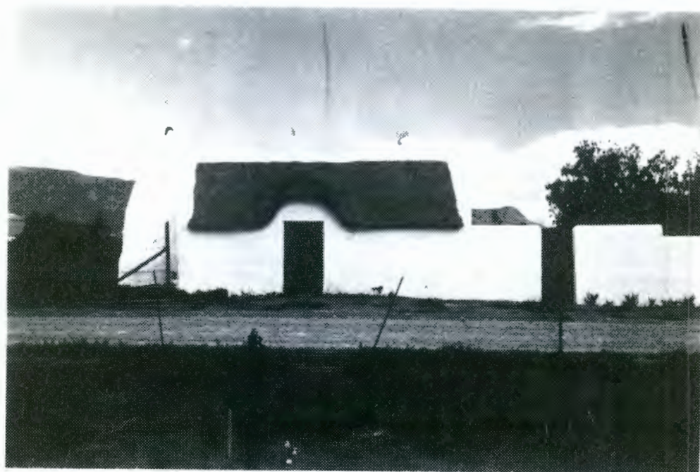
Traditional cottage with thatched roof with hooded gable over stable door. Straight end gables and external hearth. High, plastered wall adjacent, with door. No windows in street facade.
