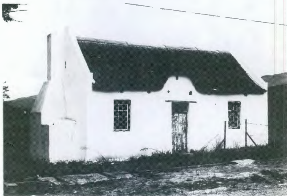
Vernacular cottage with reed thatch, straight end gables and hooded gable above door. External chimney and oven. 12-pane casements, door with fanlight and exposed wooden lintol.
