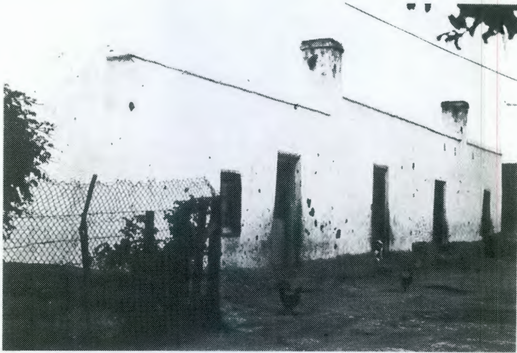
Row of parapeted cottages with two chimneys. 6-pane casements, four stable doors.
