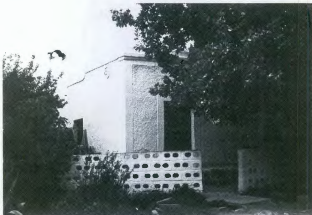
Vernacular cottage with stepped-up parapet, cornice and external chimney. Rough-plastered, with smooth plaster surrounds to openings. Stable door with 4-pane fanlight.
