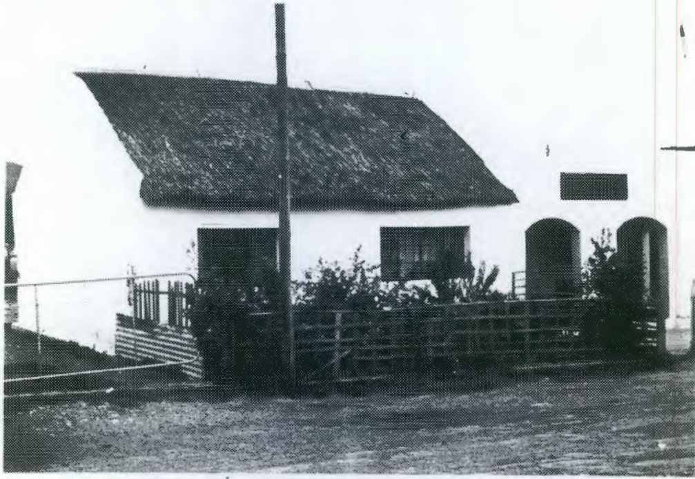
Vernacular cottage with reed thatch and straight end gables. Steel windows. Extension with stepped-up parapet and recessed verandah with arched openings.
