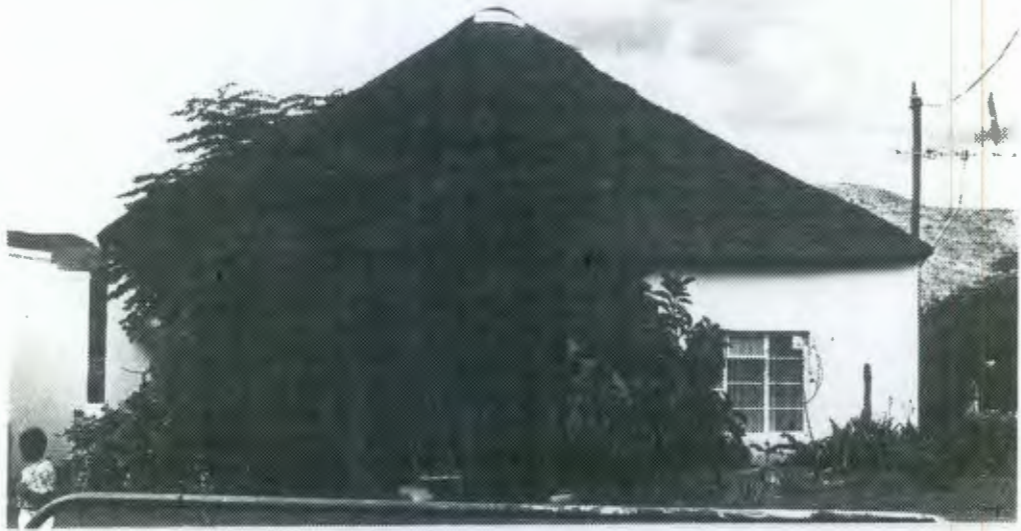
Cottage with hipped, thatched roof. Steel windows.
