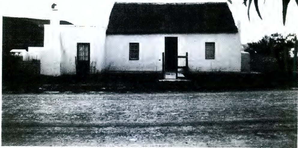
Vernacular cottage with thatched roof, straight end gables and external hearth. 6-pane casements, stable door with 3-pane fanlight. Parapeted extension with external hearth and door with window panes, projecting forward to edge of stoep.
