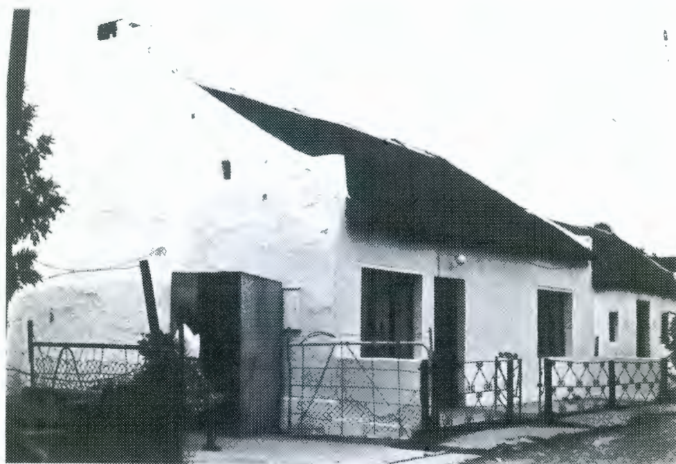
Semi-detached cottages. The one on the left has a thatched roof, straight end gables and external chimney. Modern wooden windows and stable door.
