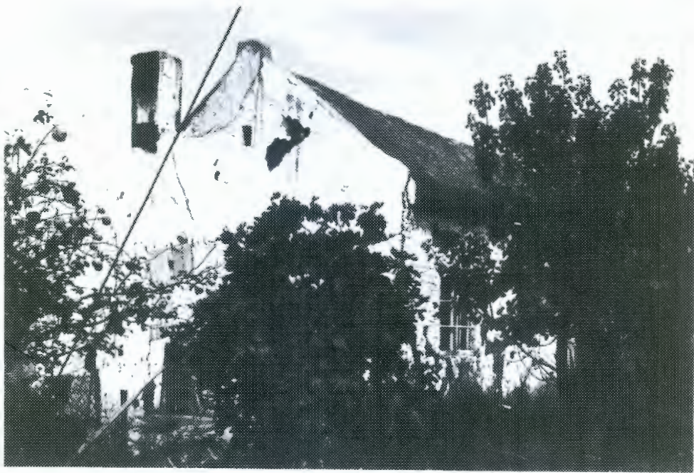
Vernacular cottage with thatched roof, straight end gables and external chimney. Casement windows.
