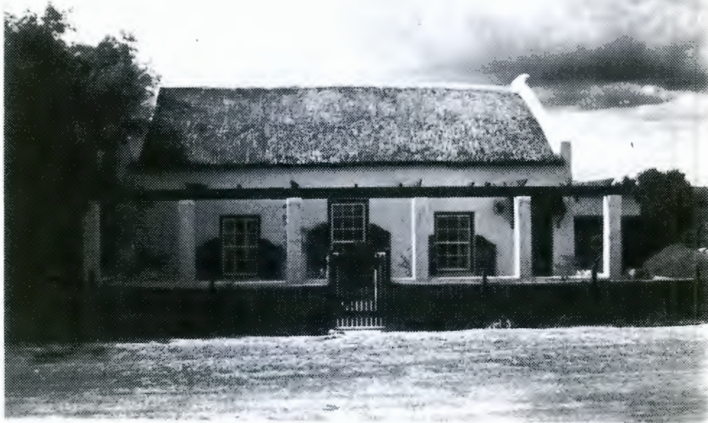
Vernacular cottage with thatched roof and straight end gables. 6 x 6 sashes and small-pane glazed door with external boarded shutters with curved tops. Stable door with canopy on wooden brackets. Pergola on plastered columns over stoep with low plastered wall. Wooden fence with gate matching shutters.
