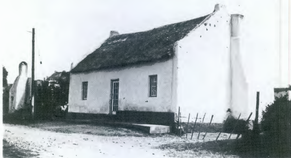
Vernacular cottage with reed thatch, straight end gables and external chimney. 12-pane casements. Small-pane glazed door.
