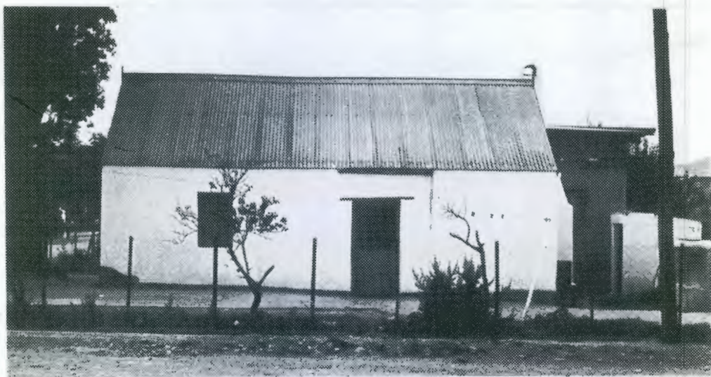
Cottage with corrugated iron roof, covered end gables and external chimney. 12-pane casement, stable door.
