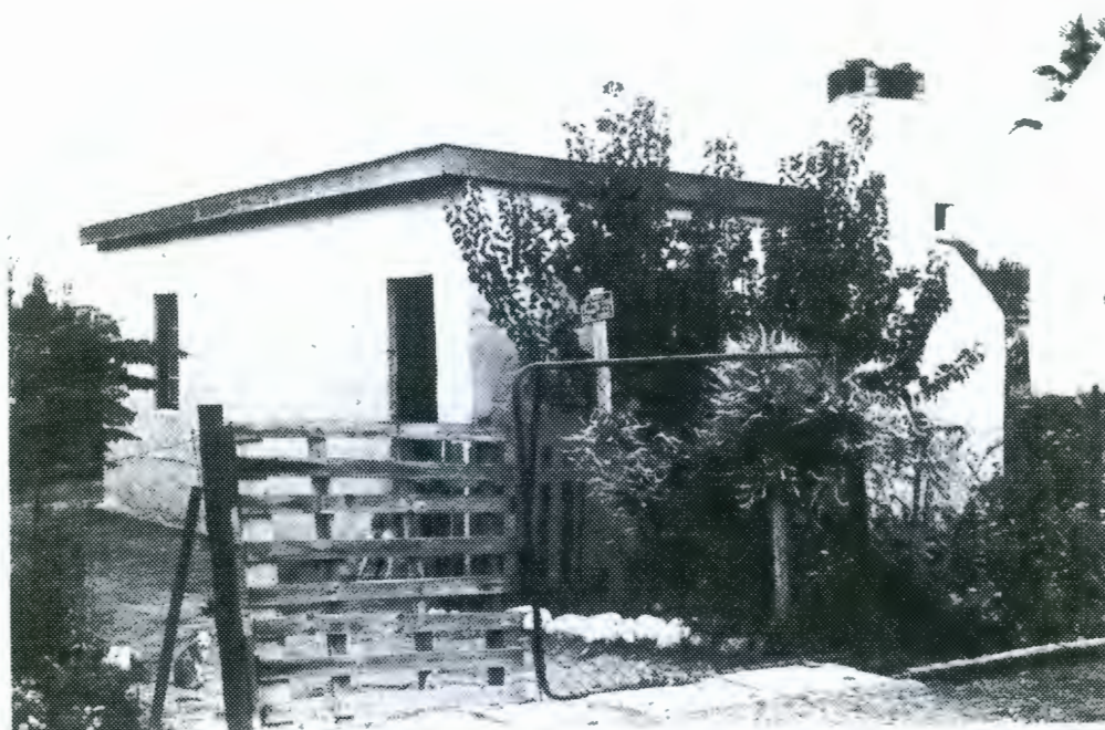
Cottage with monopitch corrugated iron roof and external chimney, Steel windows.
