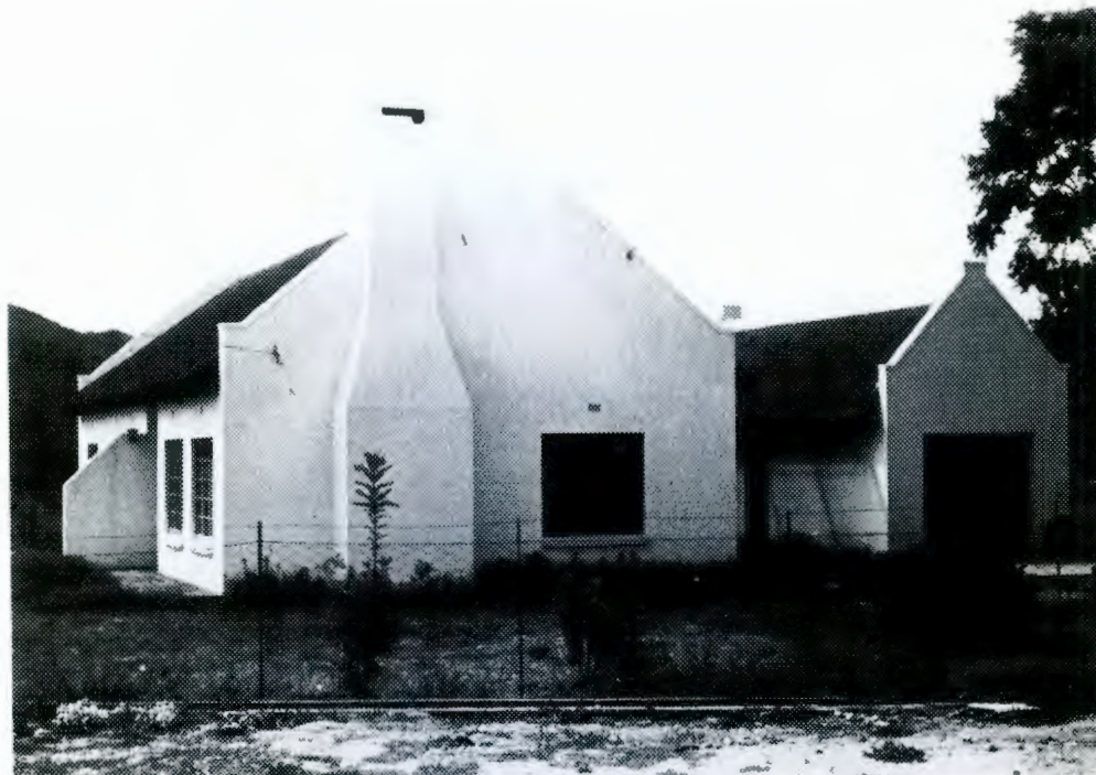
Modern vernacular style cottage with thatched roof with deep overhang, straight end gables and external hearth. 10-pane triple casement windows. Adjacent thatched garage with straight end gables.
