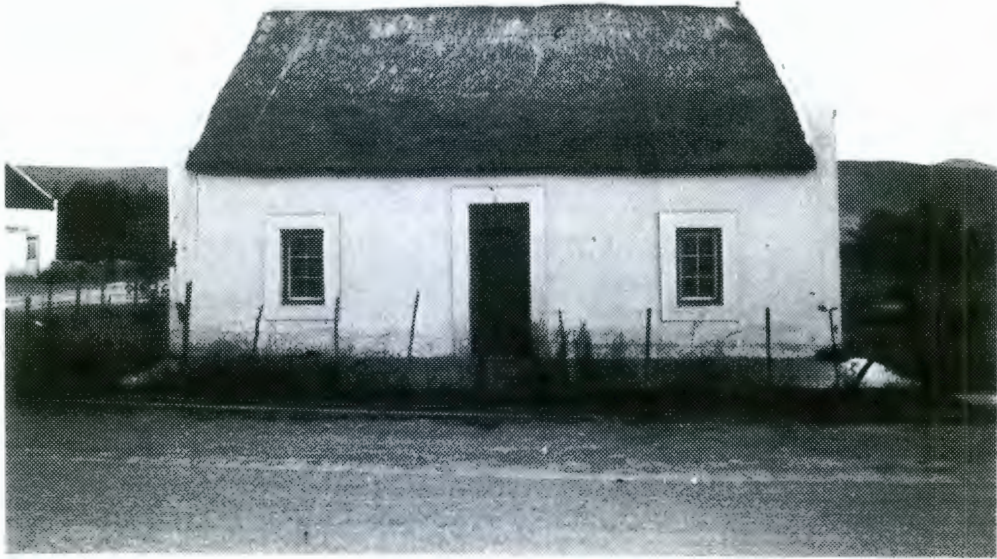
Vernacular cottage with reed thatch, straight end gables, internal chimney and off-centre loft door. 6-pane casements and stable door with fanlight, all with plaster surrounds.
