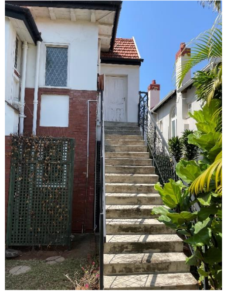
Figure H: Existing staircase to be demolished. →
