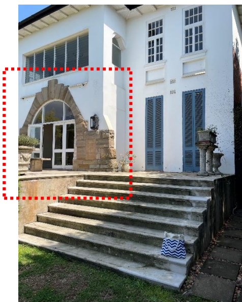
Figure L: Stone detailing. Safety railing proposed.
