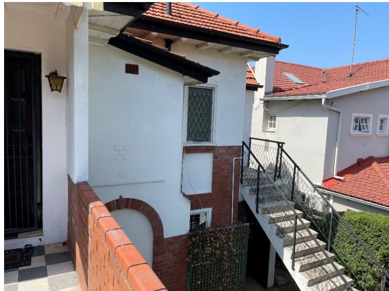
Figure D: External staircase to be demolished.
