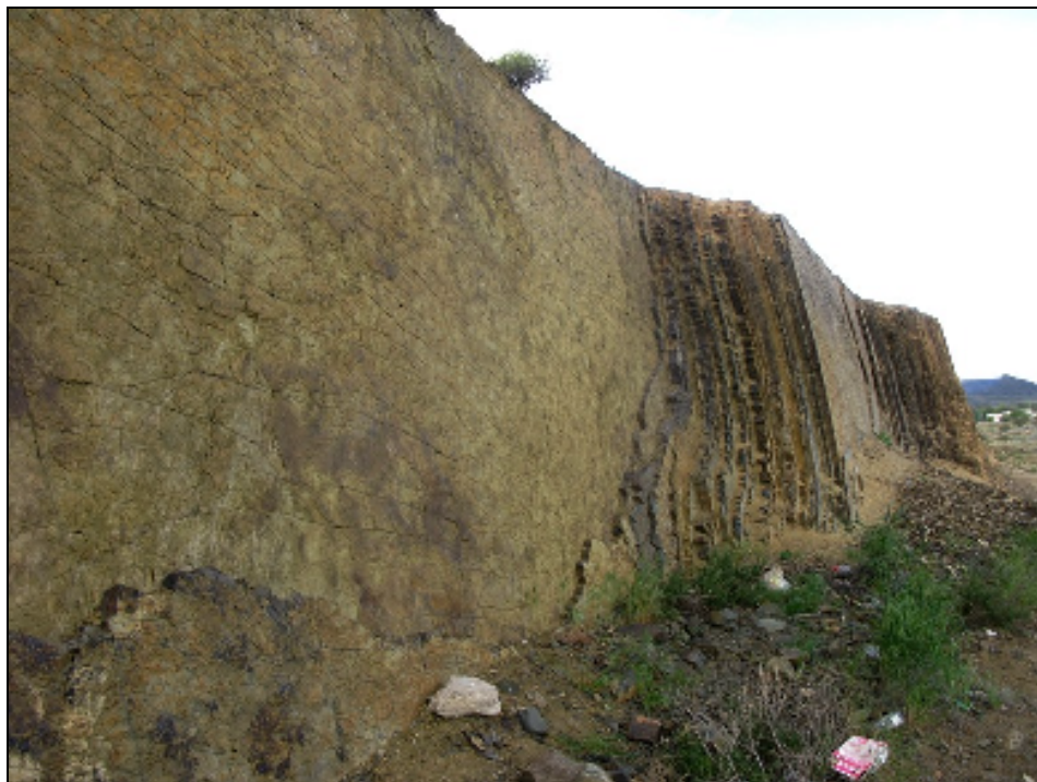
Fig. 9. Tabular, subvertical beds of the Collingham Formation exposed along the northern face of the existing DR01725/0.6/0.02R pit. The succession comprises alternating beds of silicified mudrock and pale yellow, crumbly tuff (volcanic ash).
