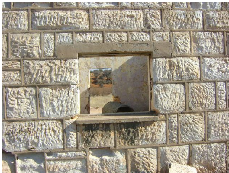
Limestone building blocks in a deserted farmhouse north of Kuruman
