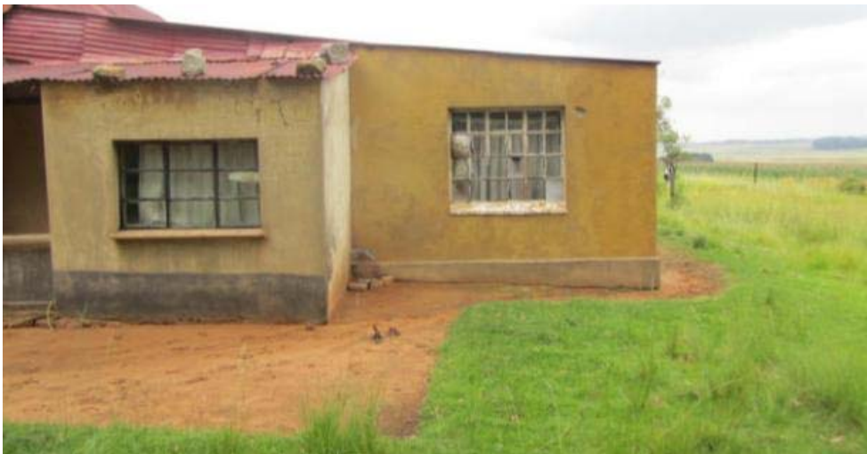
Figure 054. Close-up of the western elevation showing 'old' adaptation of veranda space and 'modern' addition. (P11)
