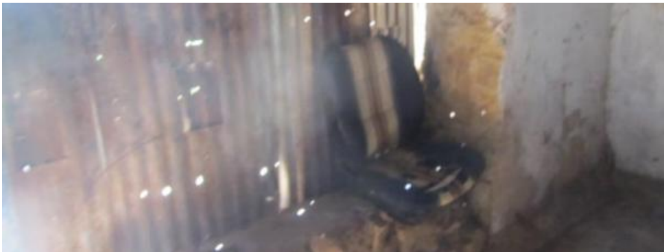
Figure 152. Original door frame of wagon shed was removed and opening is temporarily closed –up with corrugated iron. The original threshold is covered with modern masonry for unknown purposes.(P44)
