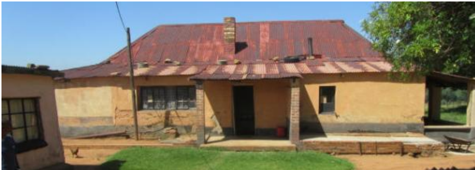
Figure 056. North elevation of house no. 1 (P13)
