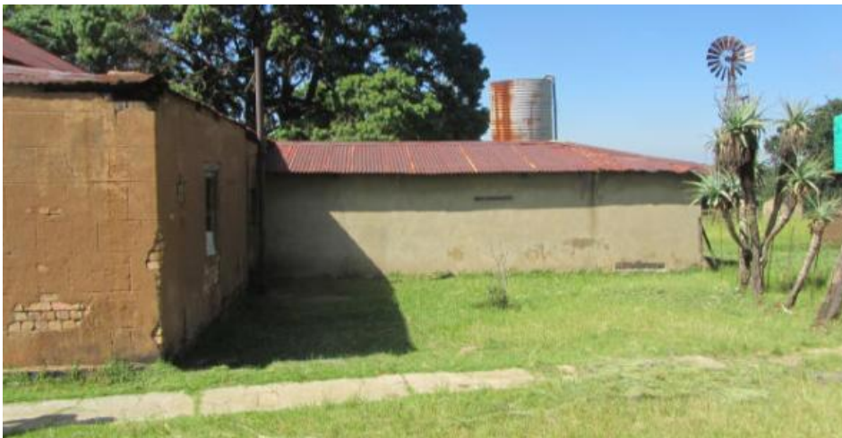
Figure 171. North elevation of the garage.(P117)
