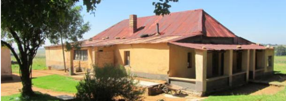
Figure 055. North-western elevation of house no. 1 (P12)
