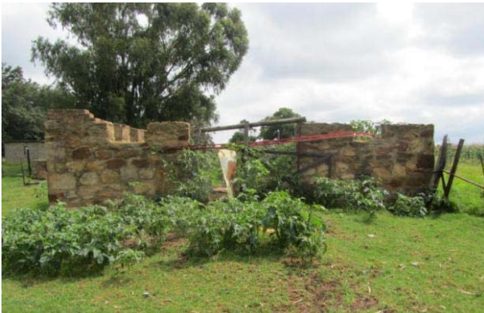
Figure 136. Southern Elevation of Milking Facility Closer inspection reveals that it is still utilised as a normal cattle kraal on a regular basis taking into consideration the build-up of dung. (P30)
