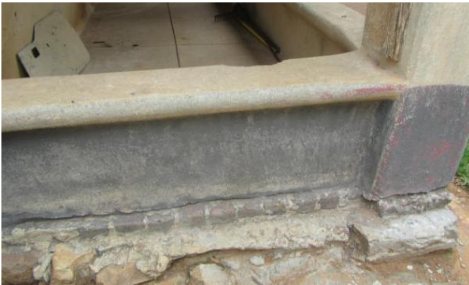
Figure 059. Detail of veranda wall and stone foundations of house no. 1. (P16)
