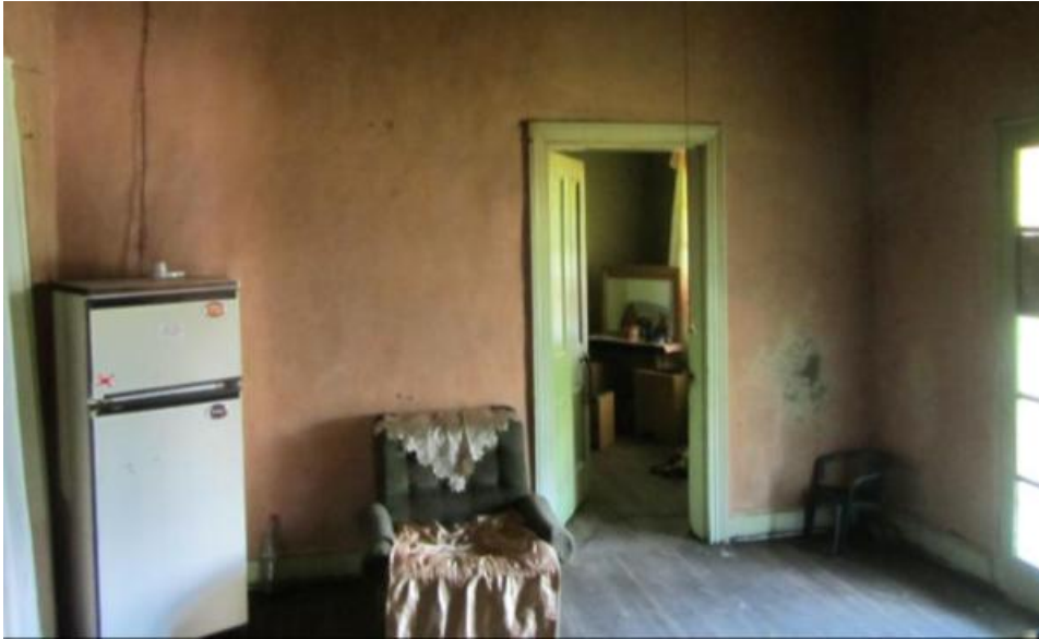
Figure 217. Note that house never were furnished for electricity, and that modern appliances are no often connected to 'roof' fittings. (P179)
