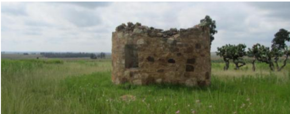
Figure 250.The fodder silo (kuilvoerput) has mostly collapsed and most of the underground section has been filled in by rubble and soil. It is approximately five meters in diameter but height and depth is unknown. On piercing of 800 wide and 1200 high occurs. Remains of a wooden frame suggest that it may have been fitted with a shutter of some kind. (P141)
