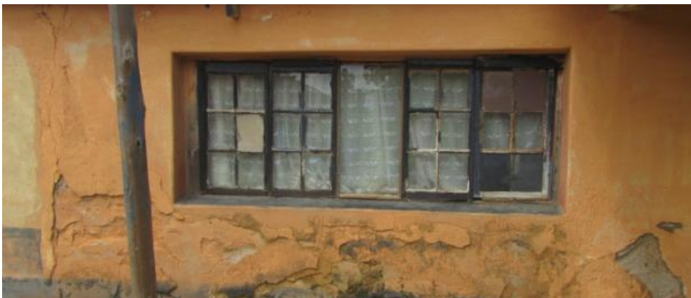
Figure 057. North elevation of house no. 1 showing detail of wooden casement window.(P14)
