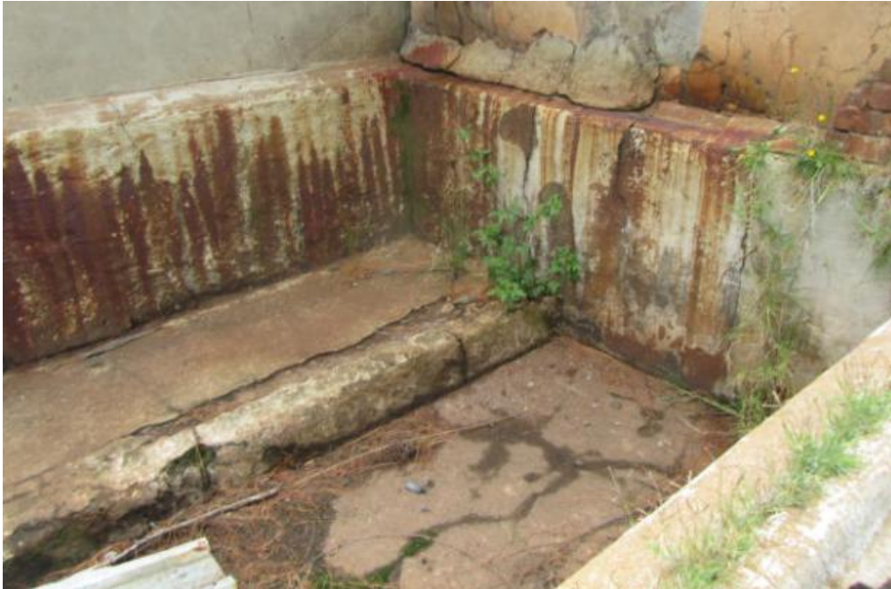
Figure 242. Interior detail of the overflow reservoir. (P133)
