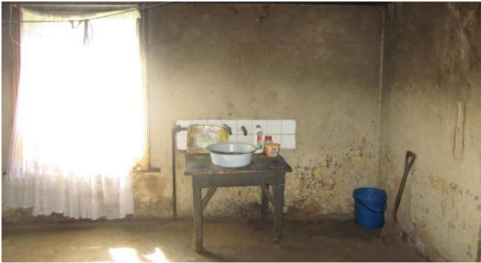
Figure 202. Basic piped water was supplied to the sandstone kitchen addition but no kitchen fittings survive. (P164)
