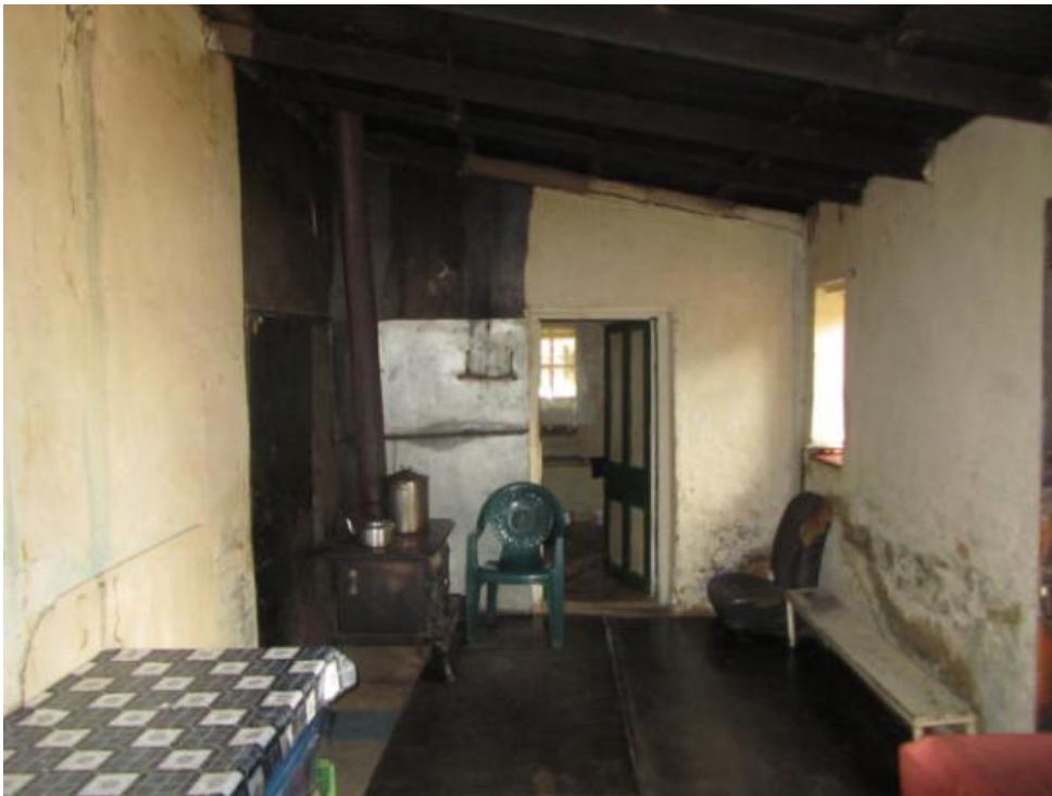
Figure 078. Westwards view in the 'kitchen' of house no 1. (P65)
