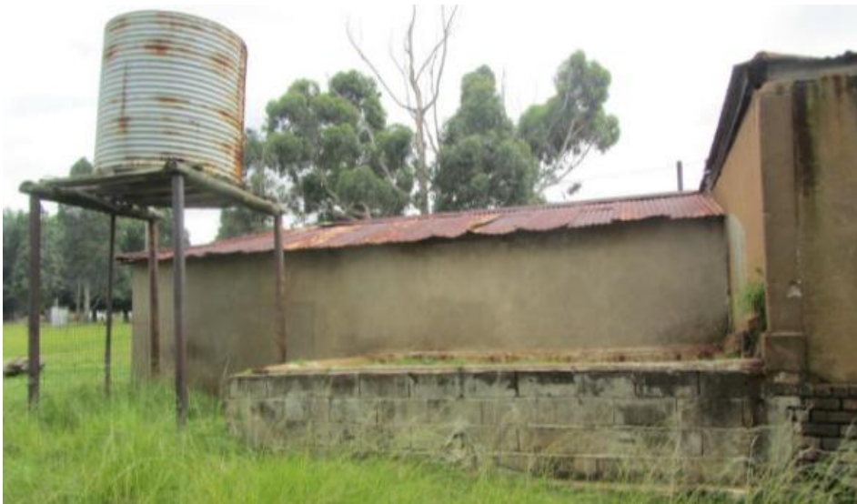
Figure241. Water overflow reservoir (swimming pool for children?) to the south side of the garage. This structure appears to predate the garage and may have been built at the time that the north eastern sandstone addition was made. (P132)
