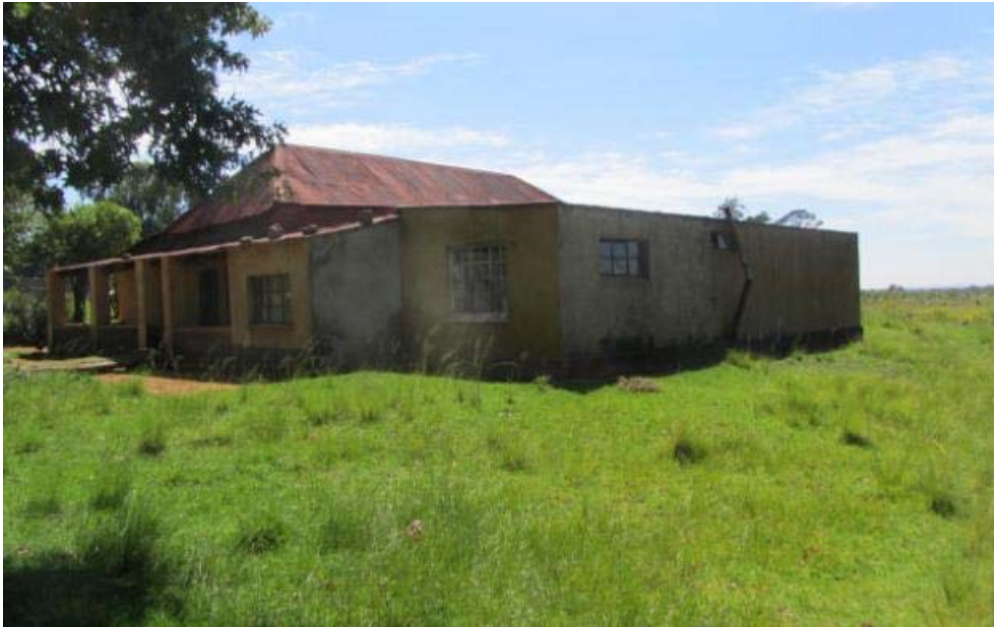
Figure 048. South-western elevation of house no.1 showing the originally adapted structure to the left and the modern addition to the right. (P5)
