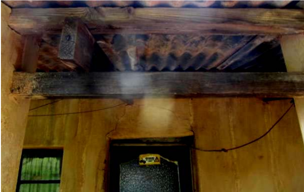
Figure 070. View of roof construction on western veranda. (P56)
