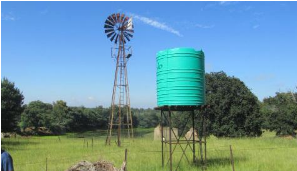
Figure 243. Original windmill and modern plastic water container. Whether these are operational is unknown as water is still collected from the fountain to the right in the picture. (P134)
