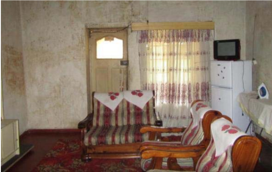
Figure 095. Internal view of door and window on the western side of the living room.(P82)
