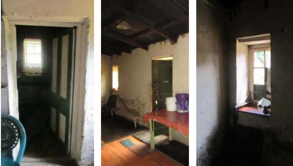
Figures 079to 081. Internal views of doors and window in the 'kitchen' of house no 1.(P66, P67 and P68)
