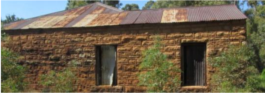
Figure 020. North elevation of the dwelling on site 4. Note presence of wooden sash windows.
