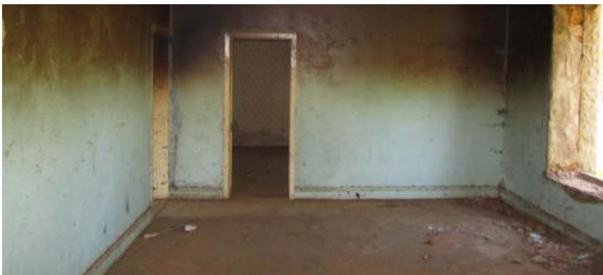
Figure 022. Although some vandalism has occurred, the dwelling is still in a good state of repair.
