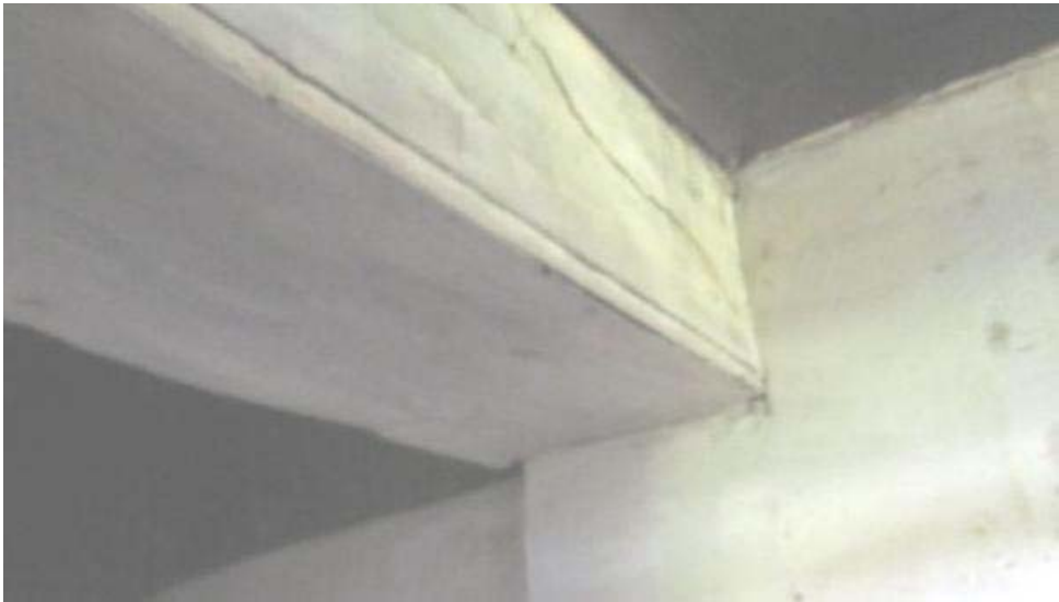
Figure 110.The beam supporting the original exterior wall.(P97)
