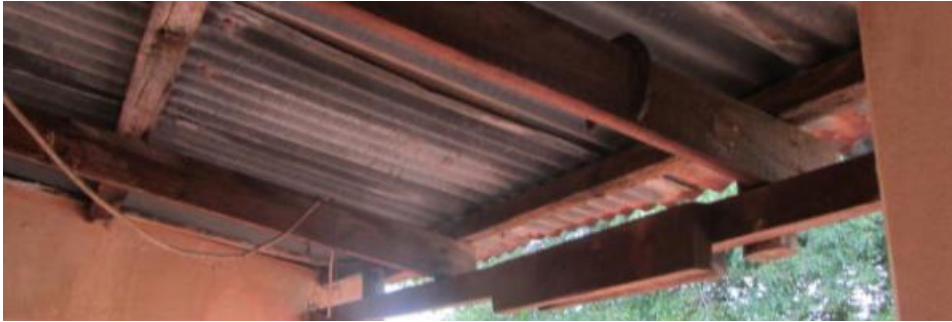
Figure 068. View of roof construction on western veranda. (P54)
