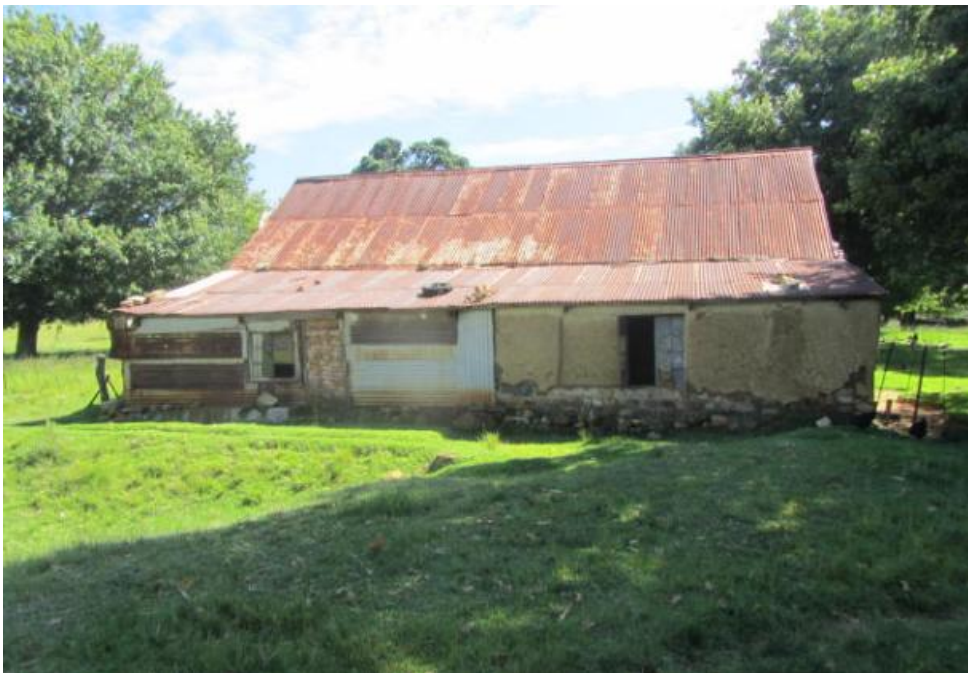
Figure 140. South elevation of the modern alterations of the lean-to on the south side of the wagon shed. (P32)
