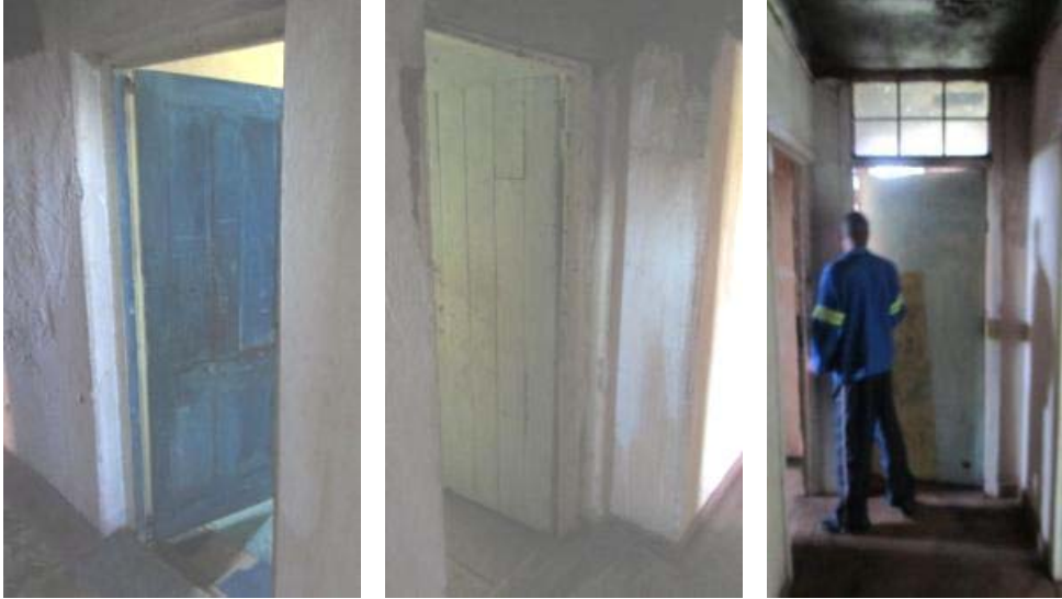
Figures 107to 109. Two doors leading to the central bedrooms and looking south along the hallway.(P94, P95 and P96)
