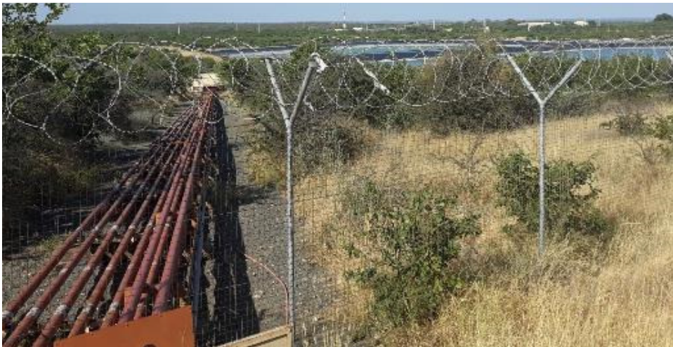
Fig. 15. Looking down on OMWSD 3 with OMWSD N&S in the background and OMWSD 3 to the right. (Photo S.M. Miller 2021.)
