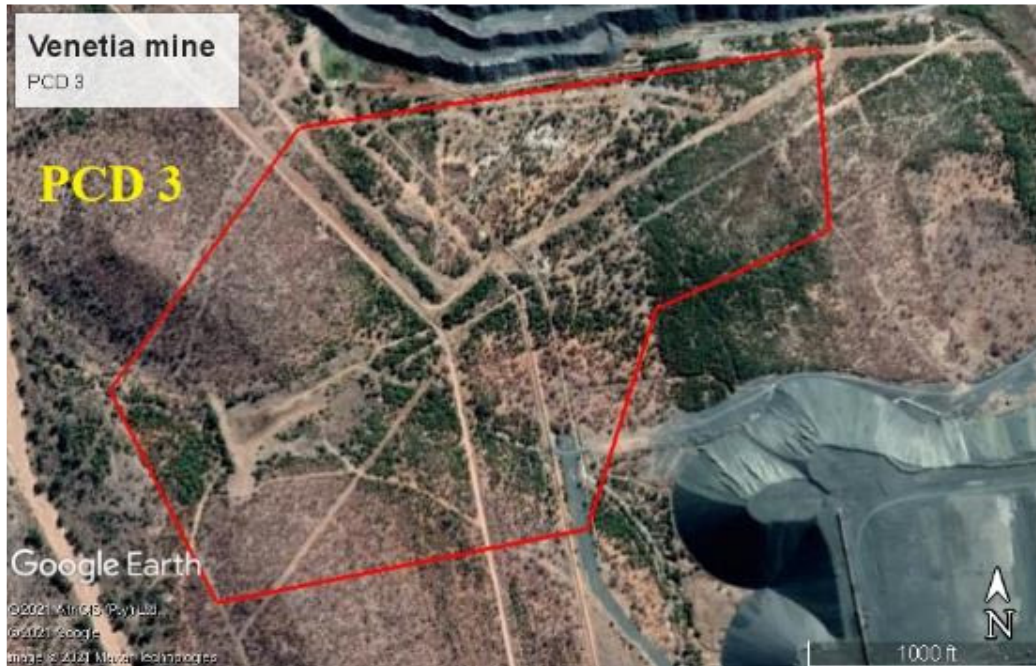
Fig. 27. This image shows the location of the PCD 3 area another proposed site for the new water management scheme. Also here can be seen that owing to 30 years of mining activity the areas are so disturbed that there is no chance for the survival of in-situ cultural material. (Google Earth 2021.) 16
