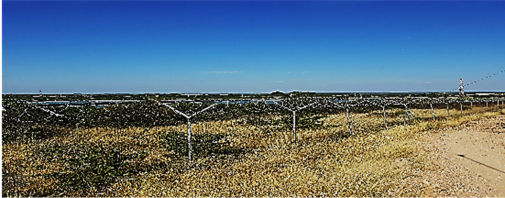
Fig. 16. Looking over OMWSD 4 to OMWSD N&S. (Photo S.M. Miller 2021.)
