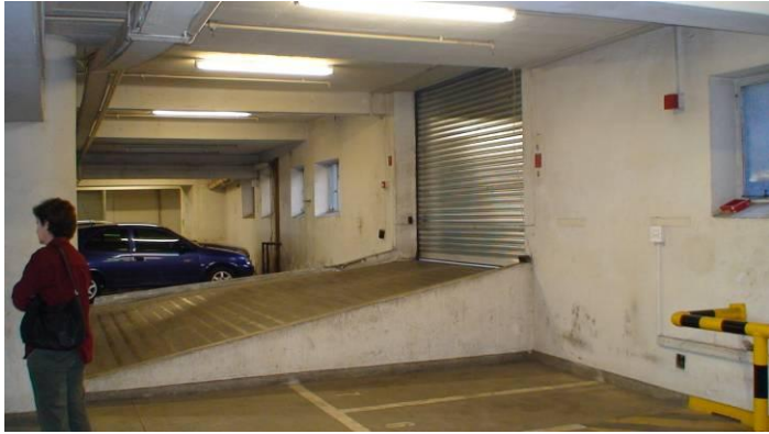
Figure 13. Basement of Provincial Government buildings has penetrated deep enough to destroy/displaced human burials.
