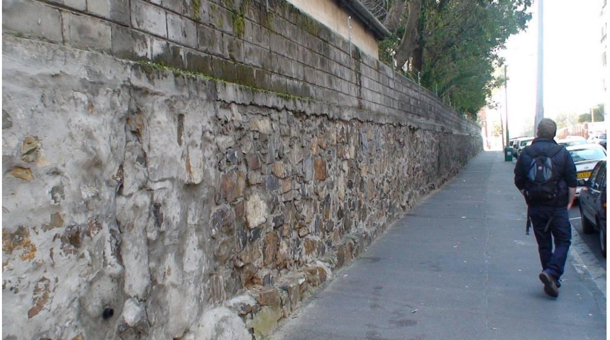
Figure 16. The old cemetery wall of the Military/Scottish cemetery is one of the oldest structures in Cape Town. Soil levels within the grounds reach the top of the bluestone wall, hence the cement block height extension.
