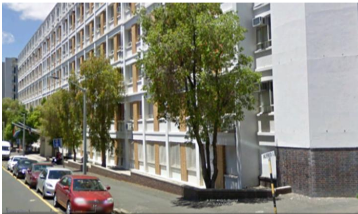
Figure 15. Provincial Government Buildings, erf 564, Alfred Street.
