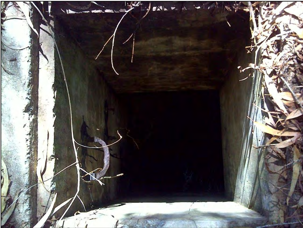
Figure 20. Looking into one of the underground open manholes.
