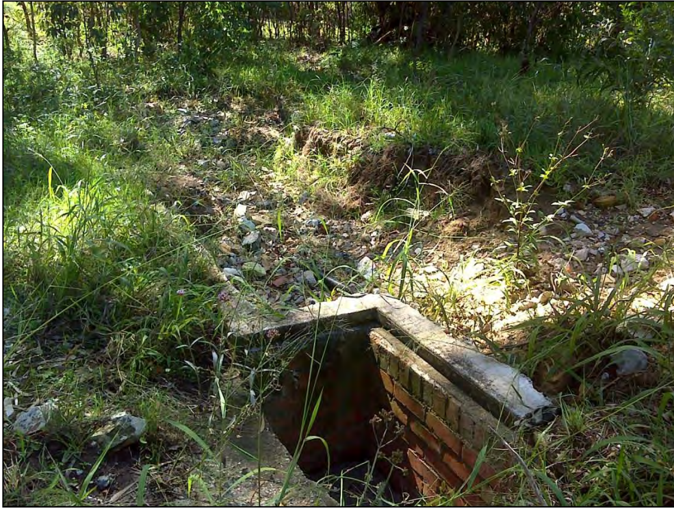
Figure 19. View of the existing underground stormwater pipeline proposed for upgrade.
