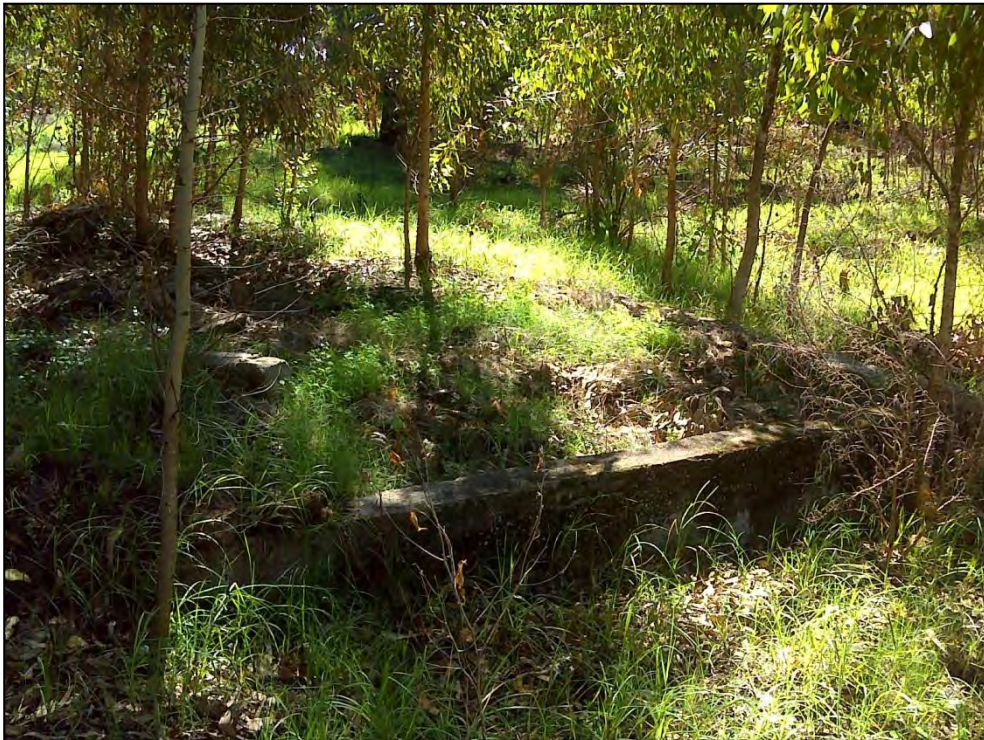
Figure 24. View of the remains of the foundations at ACSA BE1.
