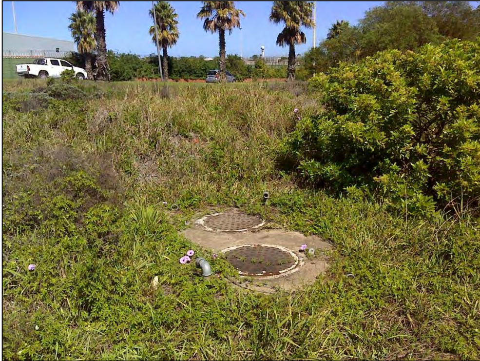
Figure 21. View of manhole covers near to Allister Miller Drive.
