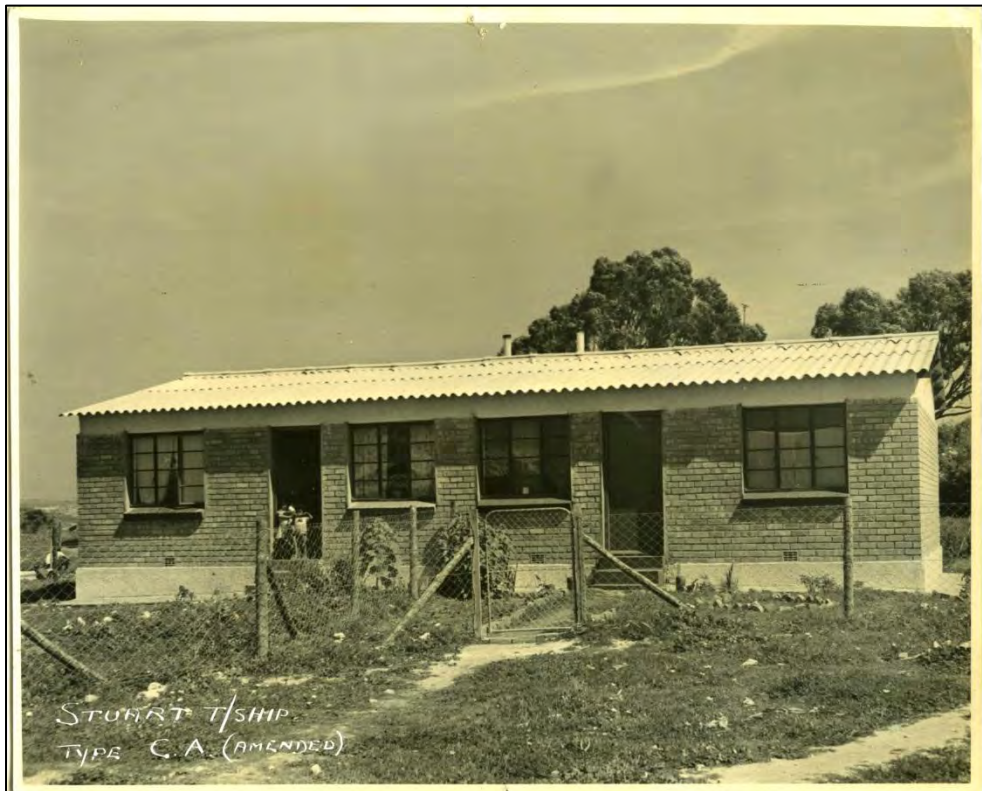
Figure 4. Close-up view of the semi-detached houses in Stuart Township (copyright Cory Library, Grahamstown).
