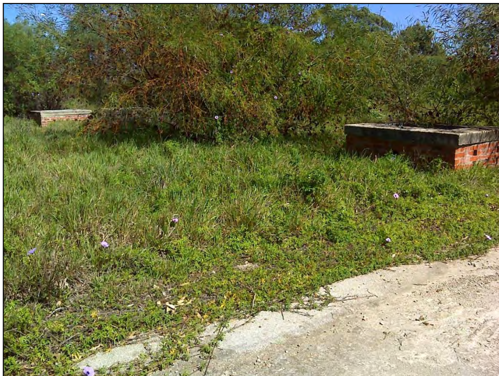
Figure 22. View the manholes for the existing stormwater pipeline.
